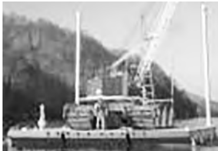
32' x 40' x 4' Sectional Spud Barge and Crane.
