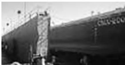
Dry Dock 220' x 70' x 6', Capacity 2800 Tons, Reported to be in excellent working condition.
