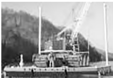
32' x 40' x 4' Sectional Spud Barge and Crane.
