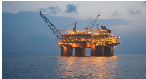
The POA pilot is underway on BP's Atlantis platform in the Gulf of Mexico. Testing is set to run to the end of first-quarter 2017. (Source: BP)
