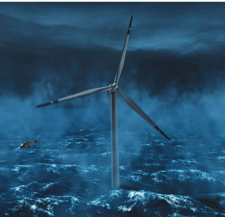
Statoil's pilot Hywind Demo steel spar floating wind turbine has been working offshore Norway in 220 m of water with no problems since 2009, supplying power directly to the Norwegian grid. (Source: Statoil)
