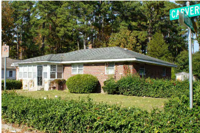
Figure 8. Ranch style residence, 1140 Carver Avenue (134-0969-0141).
