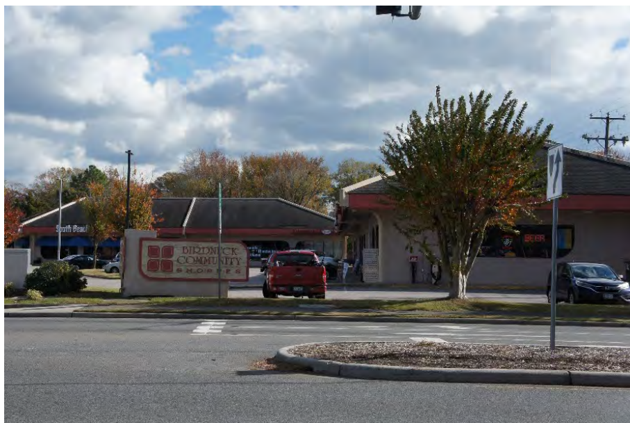
Figure 12. Birdneck Community Shoppes at the corner of South Birdneck Road and Norfolk Avenue (134-0969-0053).
