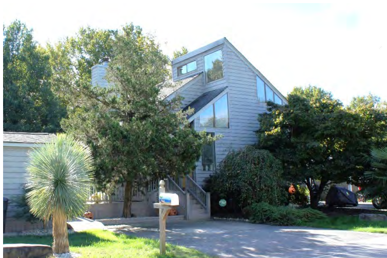
Figure 11. Example of modern infill, 148 Sea Street (134-0969-0087).
