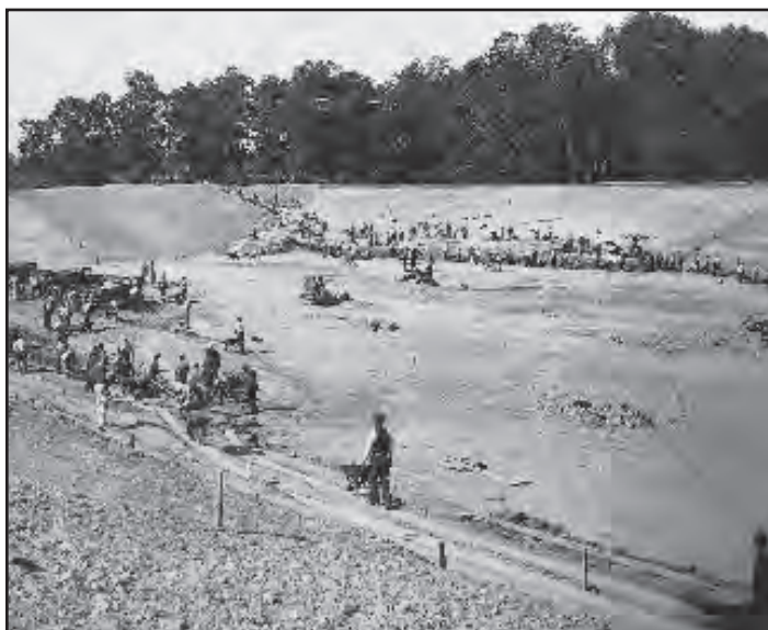
The Glass Bowl was dug out by hand by WPA workers in 1936.
