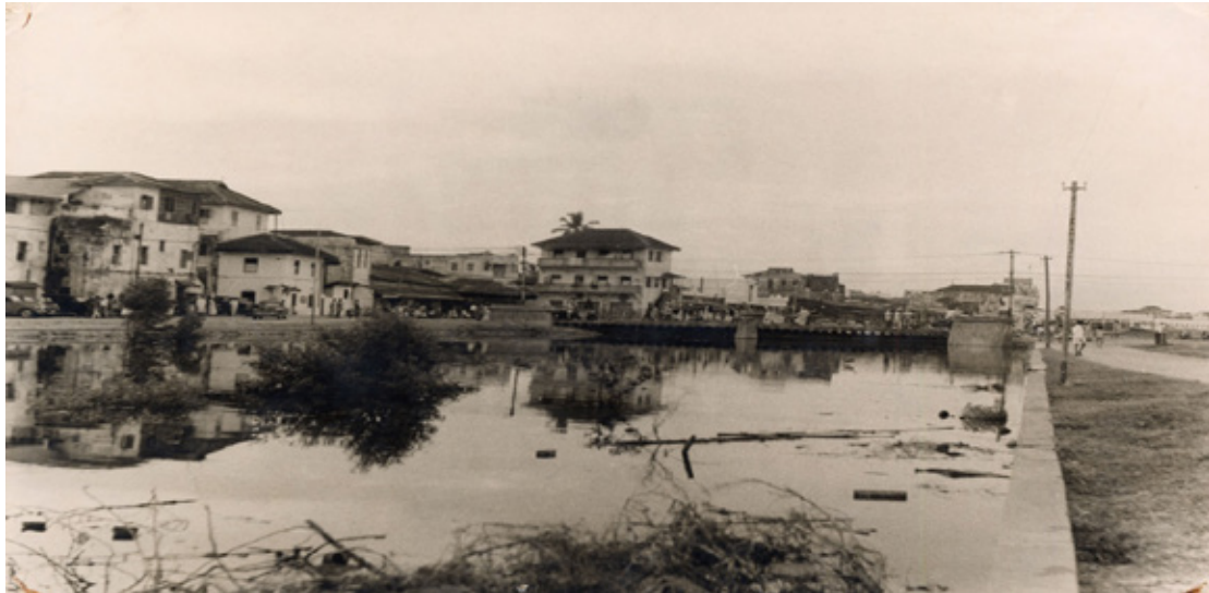
Figure 16 The Creek being filled at Darajani, photograph taken in 1943. (source: Issa 2009: 219).
