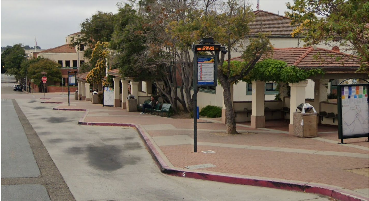
Figure 70: On-street sawtooth bus bays to facilitate on-street passenger transfers (San Luis Obispo, top , Fredericton, Canada, bottom )
