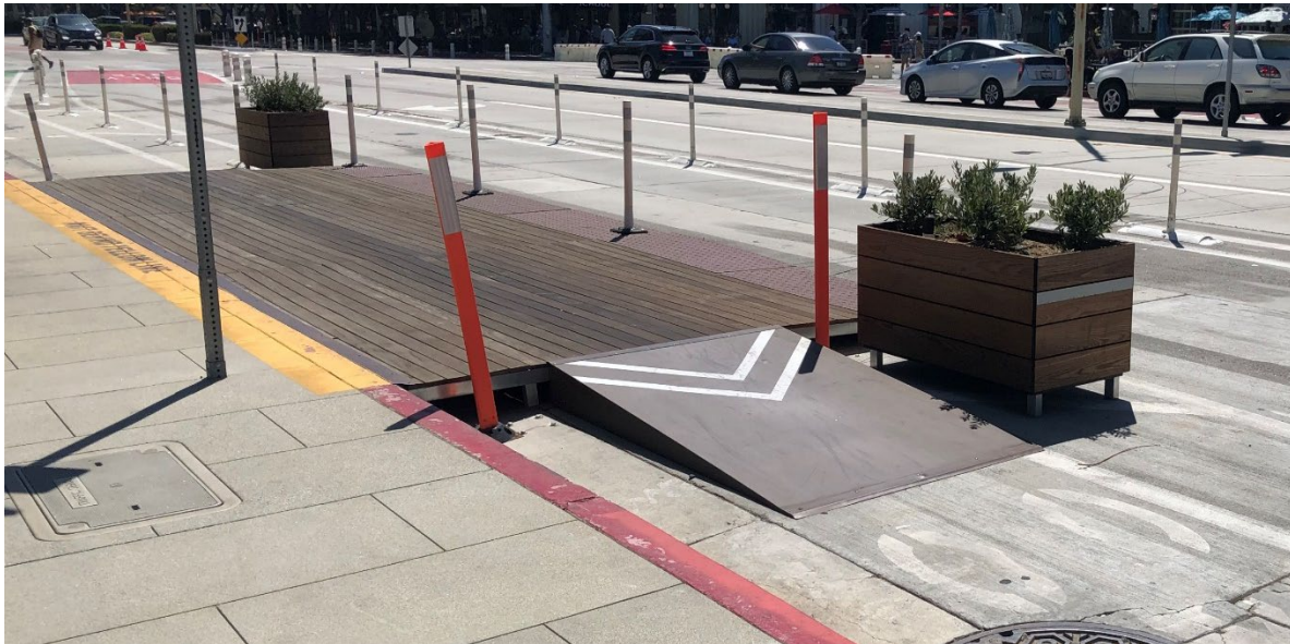
Figure 67: Bus platform through bike lane in Culver City, California
