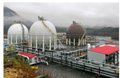
Pembina's new export facility is best viewed as a small-scale rail terminal, moving LPG from rail cars to vessels destined for international markets.
