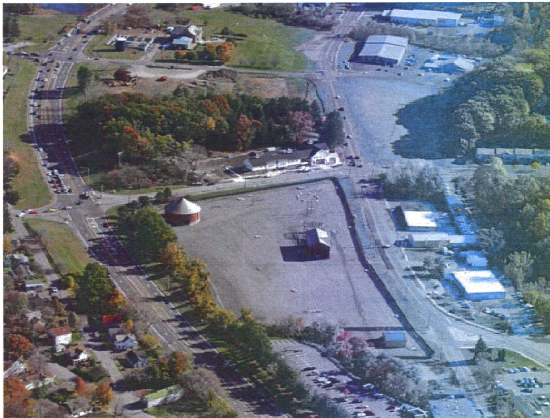
Areal Photo – Niagara Mohawk Power Corporation, Former Saratoga Springs, NY MGP
