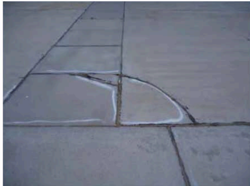
Photograph 26: Newly repaired areas marked by spray paint.
