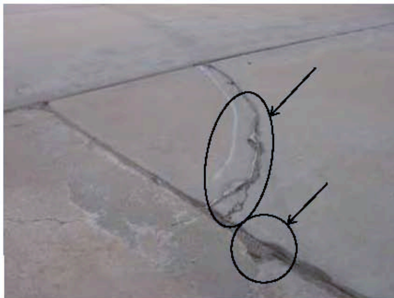
Photograph 6: A previous repair that may warrant additional repairs due to additional cracking and spalling present adjacent to the repair.
