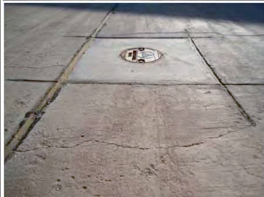
Photograph 33: Crack in concrete near monitoring well that will be monitored during the next cap inspection.
