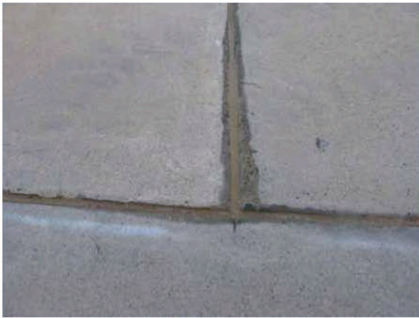
Photograph 16: Example of expansion joint in good condition.
