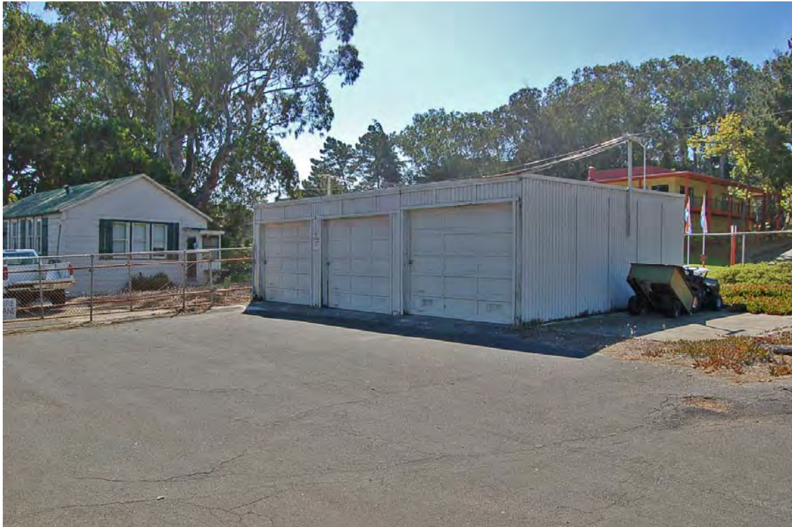
Photo 32. Garage; view to SE (D. Bradley, September 2013).
