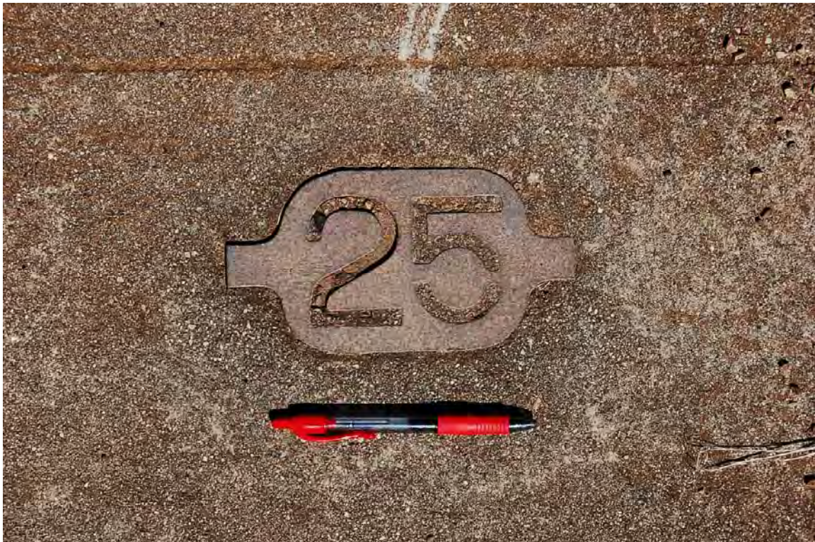
Photo 25. Detail of embedded metal tag yardage markers shown on the paved lane in Photo 24 (D. Bradley, September 2013).
