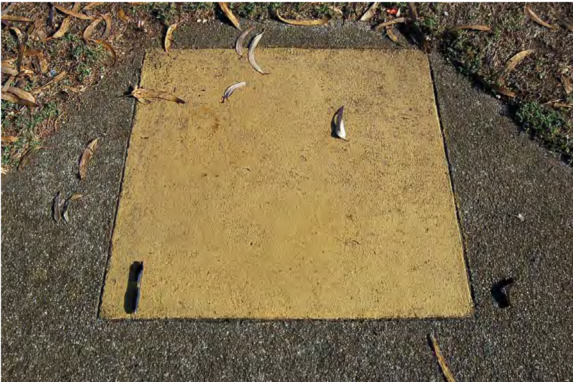
Photo 39. Detail of incised station layout on concrete path (typical to Fields 8 and 9) (D. Bradley, September 2013).
