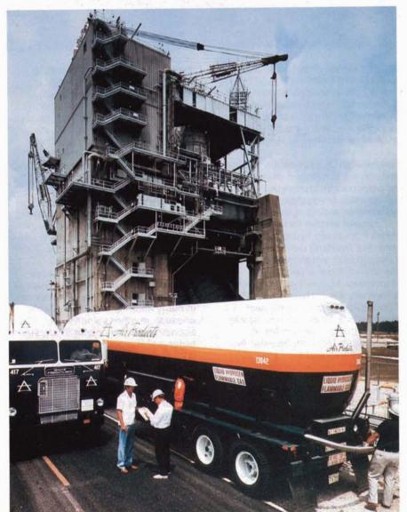
Above, a Space Shuttle engine is being tested at NASA's Mississippi Test Facility, Bay St. Louis, Mississippi. The Shuttle's main engines burn liquid hydrogen fuel supplied by Air Products and Chemicals, Inc. On a full-duration test, the engines may consume hundreds of tons of liquid hydrogen. High volume production for NASA and other government requirements gave Air Products a technology base for expansion into a variety of civil applications of liquid hydrogen.
