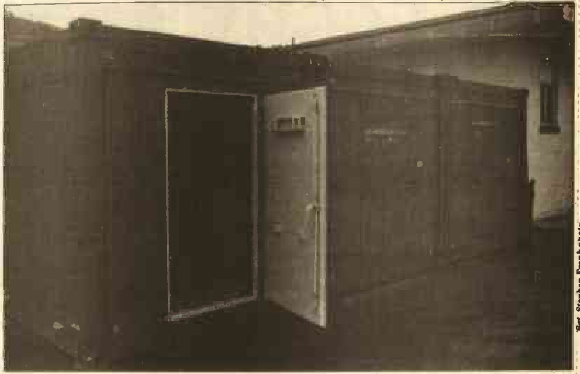
The new Marine Corps Expeditionary Shelter System, currently being tested by medical and dental units here, is scheduled to replace general purpose tents as field medical facilities.
