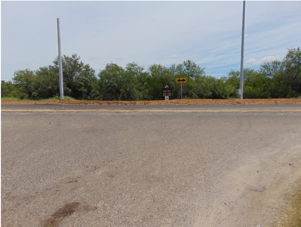
Figure 58. Project 3 DAD at Intersection of FM 3338 and Rancho Penitas Road.
