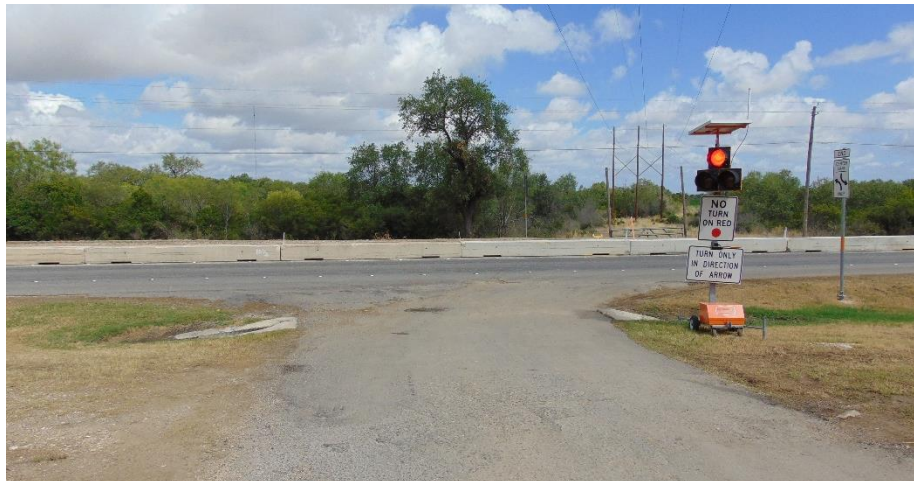
Figure 49. Project 1 DAD at Residential Driveway NB-12.
