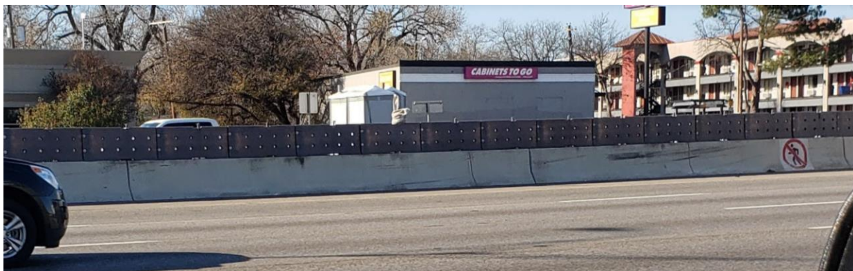
Figure 33. Stencil and Barrier on Top of Center Median on IH 35 in Austin.
