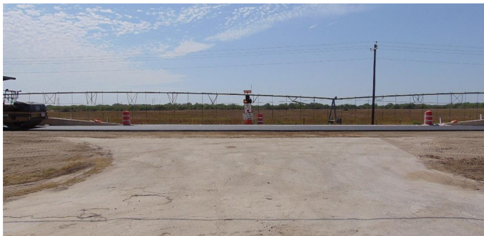
Figure 47. Project 1 DAD at Business Driveway SB-33.
