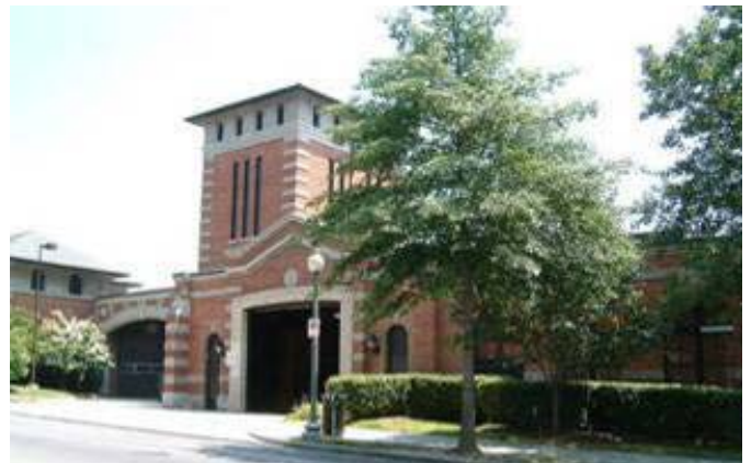
The Decatur Street Car Barn (a.k.a. the at Capital Traction Company Car Barn or Northern Carhouse), at 4615 14th Street
