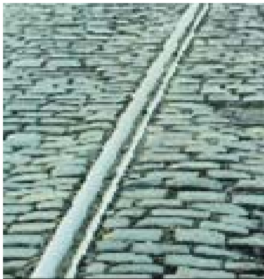
In 1852 Alphonse Loubat invented a side-bearing rail that could be laid flush with the street surface, allowing the first horse-drawn streetcar line.
