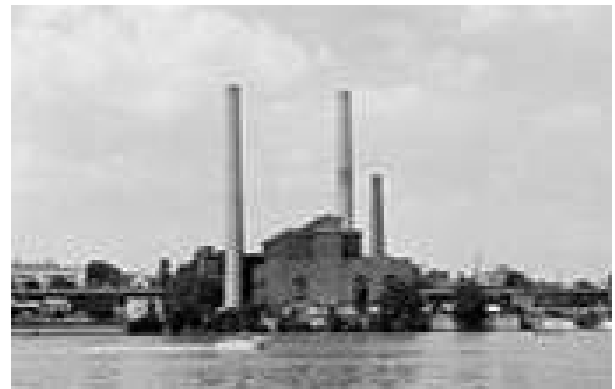
Transit Power Plant Built in 1910, Shut Down in 1935 and Demolished in 1968, Georgetown Waterfront
