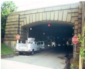
North Capitol Streetcar Tunnel, now a Parking
