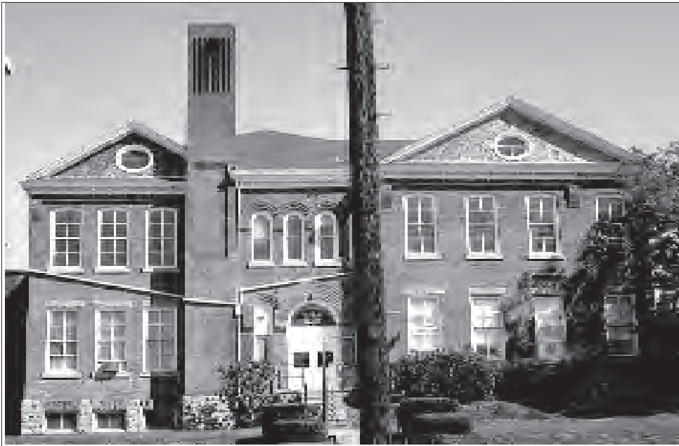
North Street Elementary School, front elevation, photo by Marie Lanser Beck
