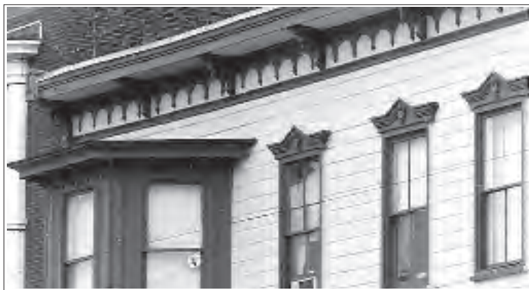
Smith Building, cornice and window details, photo by William J. Sheppard
