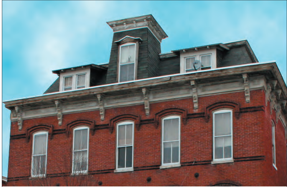
Bonebrake-Harbaugh Building, cornice detail, photo by Stephen Monn
