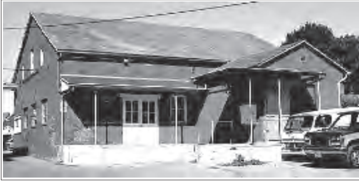
Waynesboro Ice and Cold Storage Co., Locker-Freezer Building & Office, photo by Marie Lanser Beck
