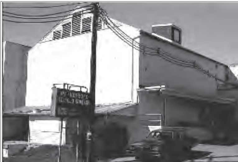
Waynesboro Ice and Cold Storage Co., Engine Room & Ice Storage, photo by Marie Lanser Beck
