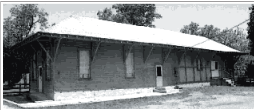
Mont Alto Railroad Station, photo by James M. Smith
