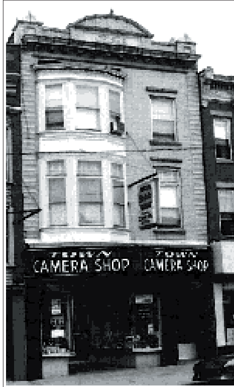
John B. Geiser Building, photo by Dan Arthur
