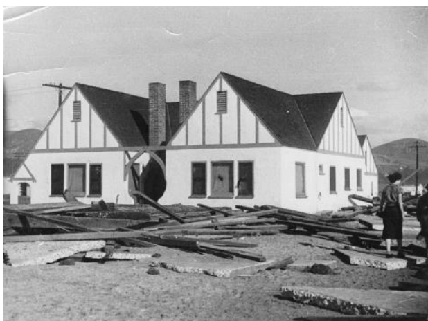
Storm damage to a Period Revival cottage on Seward Avenue, December 1937.
