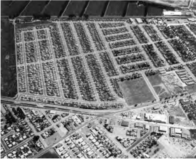
Aerial View of Five Points Park.
