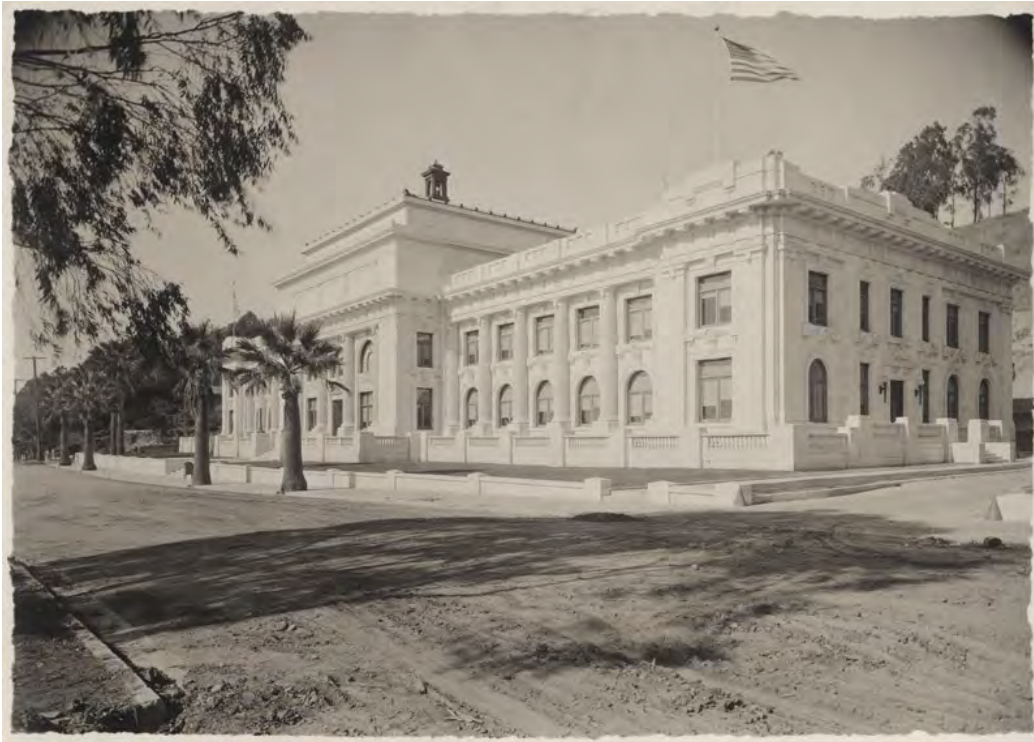
Ventura County Courthouse. Source: California State Library .
