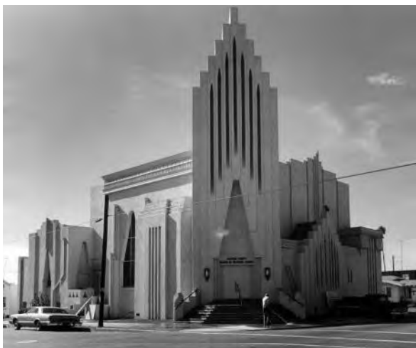
First Baptist Church, 101 South Laurel Street, c. 1975.
