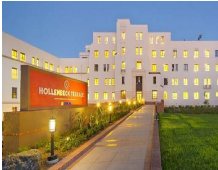
Front, Hollenbeck Terrace Apartments
