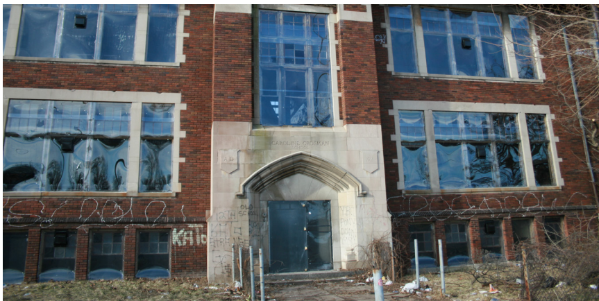
Crosman Elementary School, 2017
