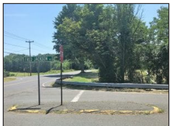
Construction will begin July 8 on this culvert at the corner of Fred Jackson and Granville roads.
