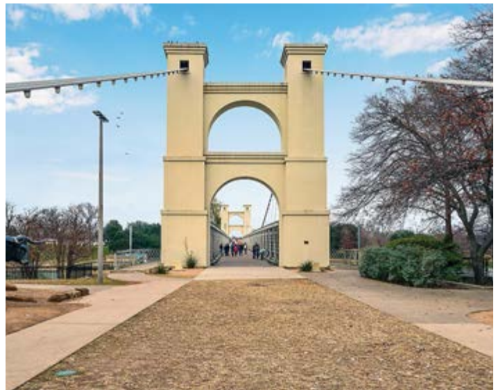
The famous Waco suspension bridge was first opened January 7, 1870 as a private toll bridge over the Brazos River for cowboys driving cattle on the Chisholm Trail. At that time it was the longest (475 ft) single span suspension bridge in the world. Many years later the county bought the bridge and turned it into a pedestrian and biking thoroughfare.
