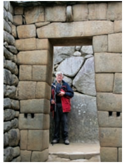
Entrance gate to the Palace of the Princess and Temple of the Sun
