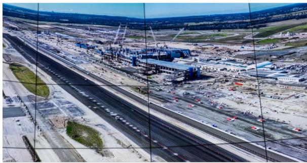
Current construction. The runway is 3 km long and fill from the road tunnels that were being bored for the Sydney road system were used as the substrata for the runway
