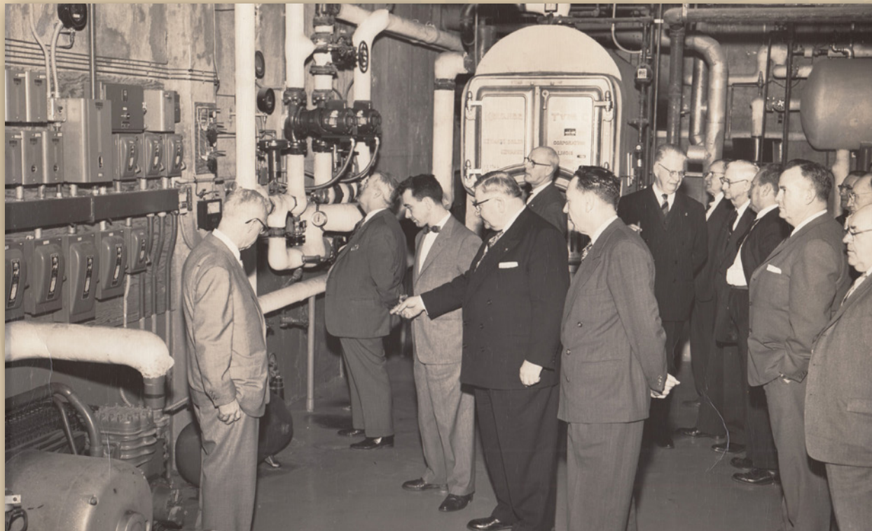
The United Association's National Apprenticeship Committee inspects the Local 562 Training Center in its union hall at 1242 Pierce Avenue in 1959.
