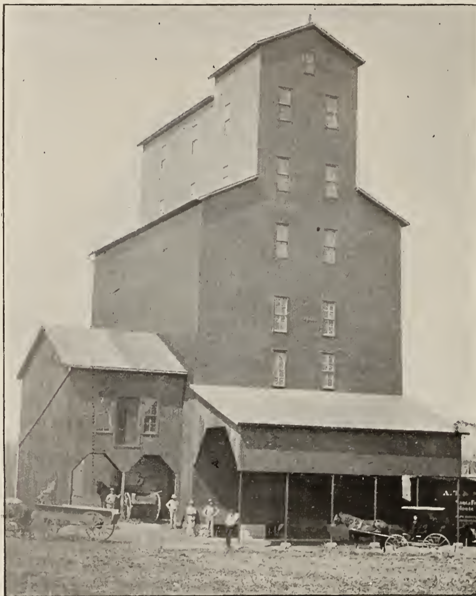
NEW ELEVATOR AT WELLINGTON, KAN.
