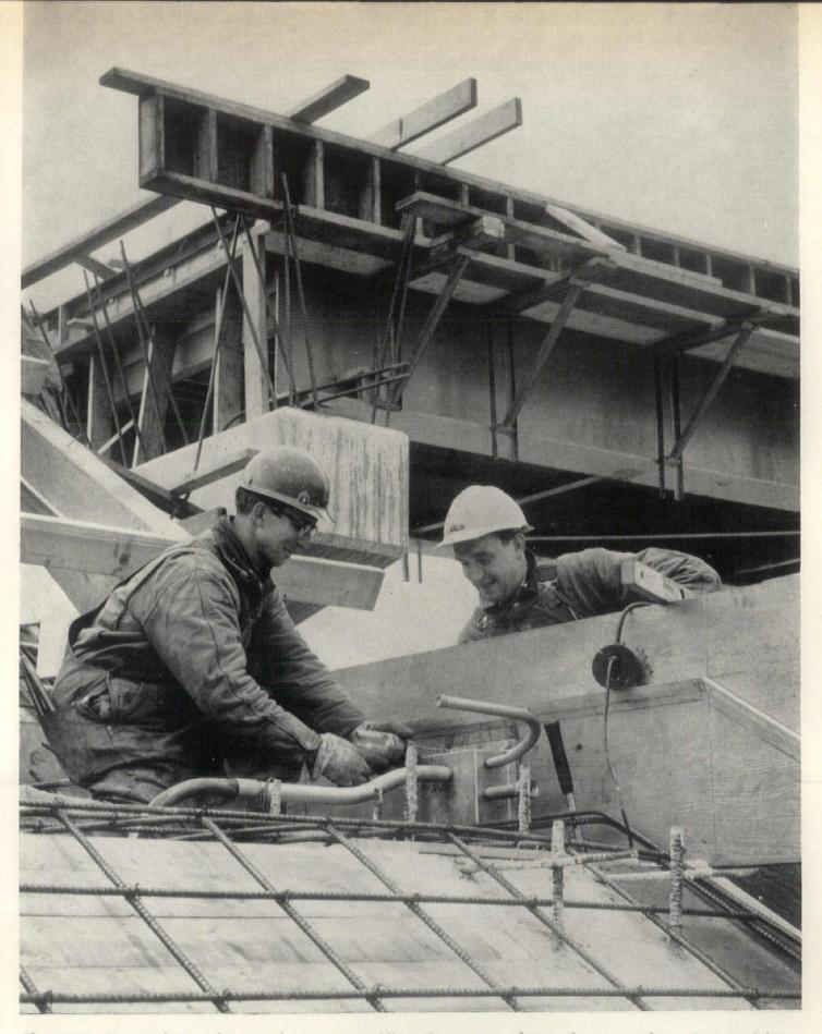
Electrician Howard Lamphier and apprentice Nino Como are shown here roughing in provisions for electric heating cables which will keep the tournier pedestrian bridge over the Southfield Expressway free from ice and snow.
