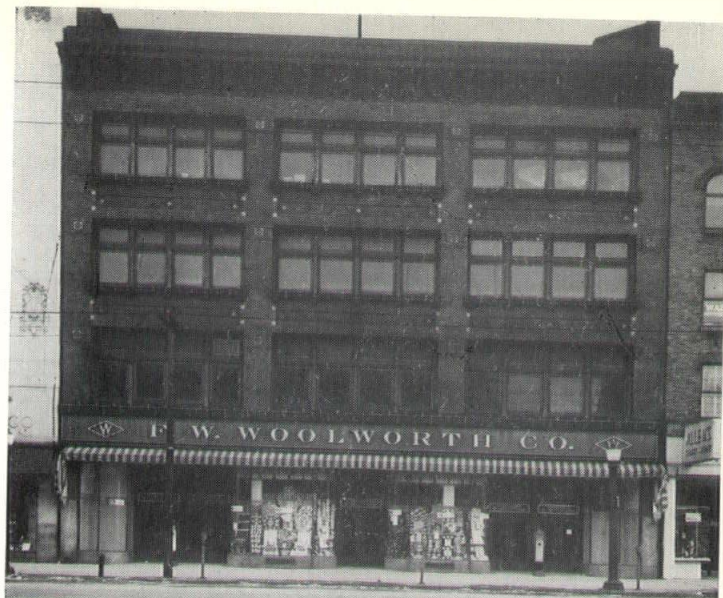
BEFORE — The F. W. Woolworth Co. Building before remodeling
