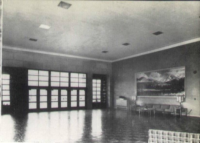
Main entrance of lounge-lobby. The ceiling is Fiber-glas acoustical tile. The floor is asphalt tile.
