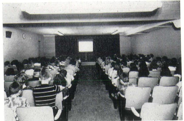
Through use of Fiberglas acoustical tile on the ceiling and with cinder block walls and asphalt tile floor, this visual education room is as quiet as a forest.
