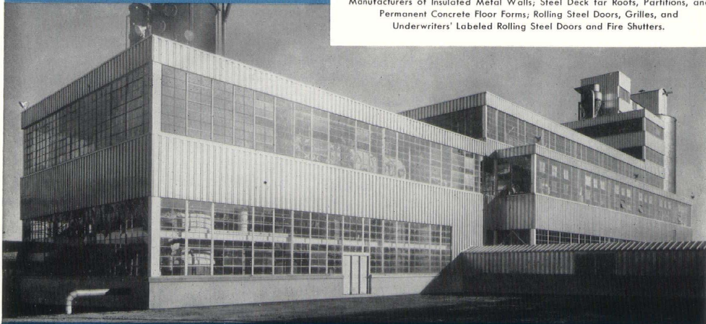
Mahon Aluminum Insulated Metal Walls and Mahon Steel Deck Roofs were employed in the construction of this new plant for Quaker Oats at Omaha, Neb. Verne E. Alden Company, Chicago, Ill., Architects and Engineers. Parsons Construction Co., Omaha, Neb., General Contractors.
