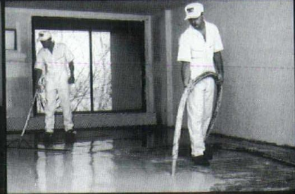
Dura-Cap ™ or Level-Right ™ can level to a smooth, hard (up to 4650 psi) underlayment.
