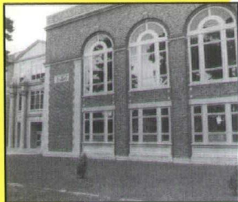
Punched Openings (West High School - Green Bay)
