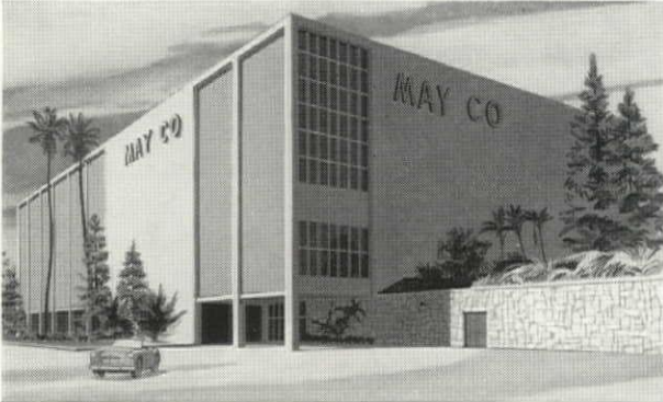
MAY COMPANY SHOPPING CENTER, WEST COVINA: Rockwin Prestressed Concrete Corporation, states, among other reasons for the choice of this method for this $12,000,000 development: "... long spans with minimum intermediate columns permitting maximum unobstructed areas... low cost and elimination of maintenance." Architect Engineer: A. C. Martin & Associates, Los Angeles; Contractor: T-S Construction Engineers, Inc., Los Angeles; Prestressed Concrete Manufacturer: ROCKWIN PRESTRESSED CONCRETE CORP., Santa Fe Springs, Calif.
