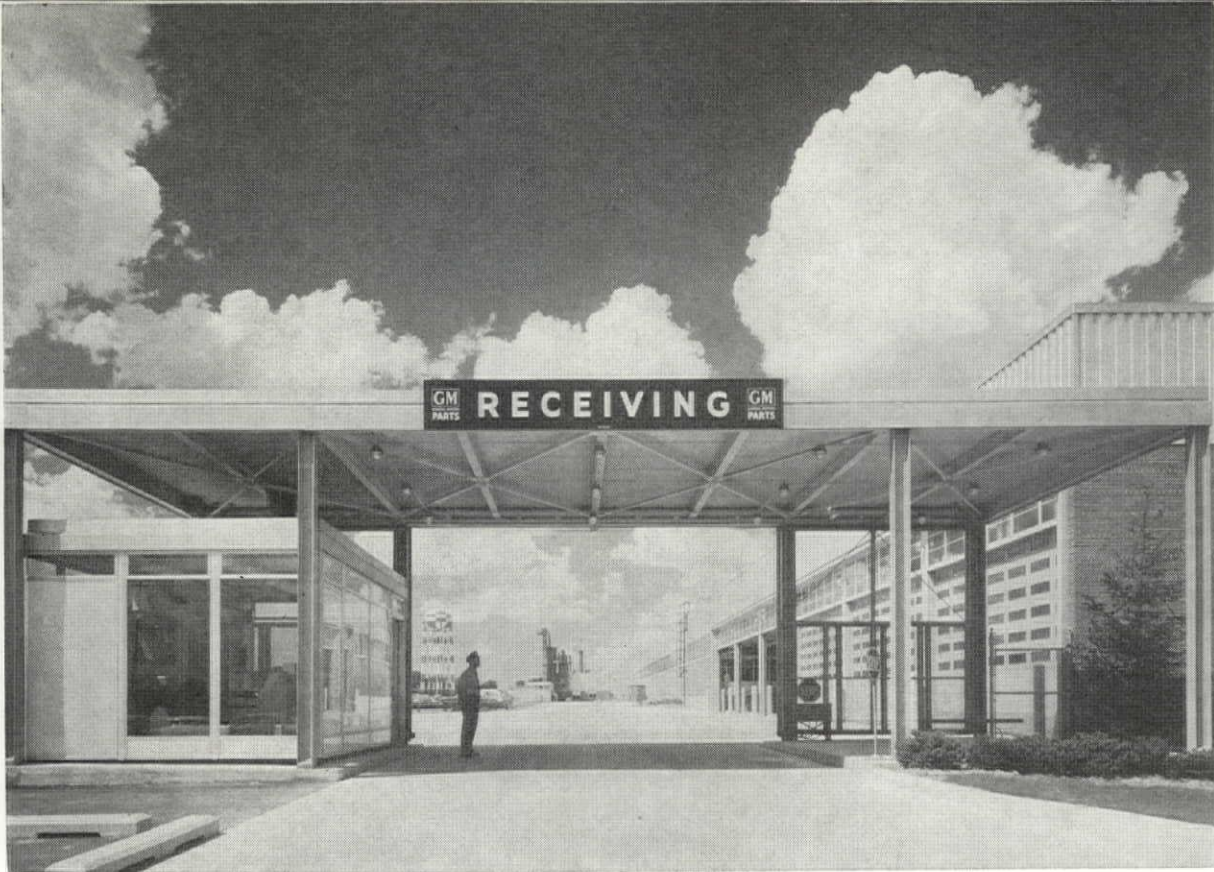
West guard house and truck shelter. Guard house, of aluminum, \frac{1}{4} " plate glass and off-white insulated porcelain enamel panels, rests on raised concrete pad beneath truck shelter supported on steel columns, painted gray. Truck shelter has exposed roof framing, exposed corrugated metal deck and aluminum fascia to match fascia of guard house.
