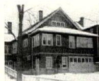
The G. L. Tubbs residence. Iron Fireman installed by Rockwell Coal Co., Pontiac.
