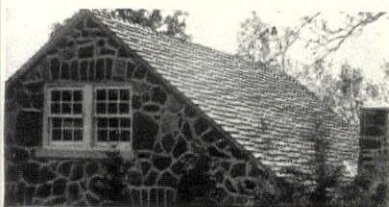
Kenmar Copper Roof at Oxford, Conn., Margery Wilson, 1148 5th Ave., N. Y.
