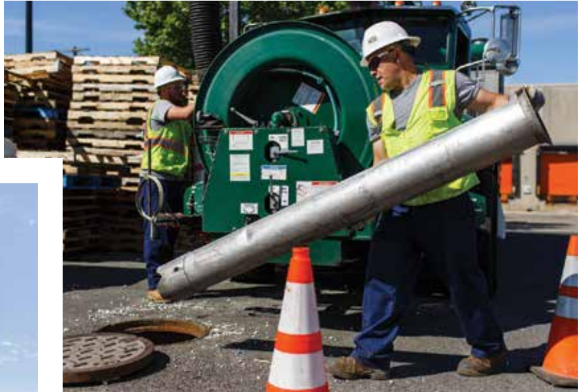
Eddie Riednger and Nelson Solares connect the extension tubes on the vacuum boom while setting up for a cleaning job.
