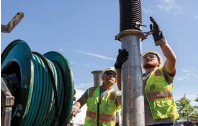
Eddie Riednger and Nelson Solares connect the extension tubes on the vacuum boom while setting up for a cleaning job.
