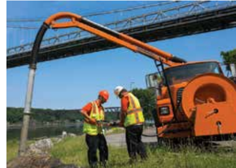
Below: The Angelo brothers vacuum out a catch basin near the Mid-Hudson Bridge in Poughkeepsie, New York.
