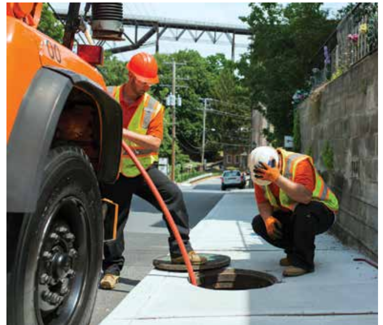
Chris (left) and John Angelo clean out a catch basin in Wappingers Falls, New York.
