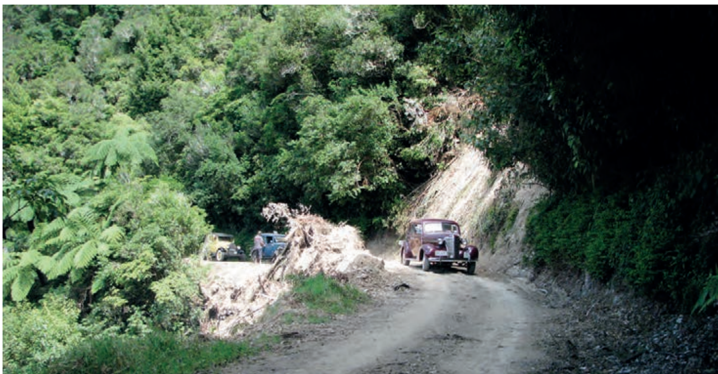
Wellington: Slip on the Motu Road.
