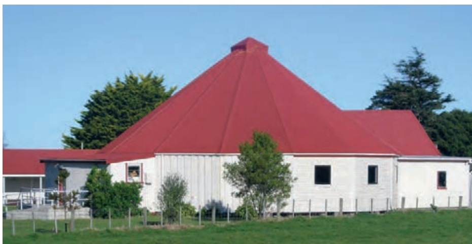
The Rongo Mai Wahine marae at Mohaka, which was built from pit sawn timber in 1885.
