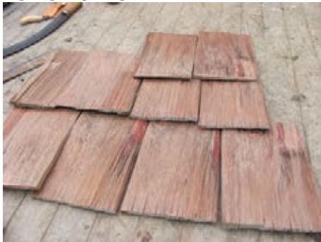
Horowhenua: Finished shake shingles.
