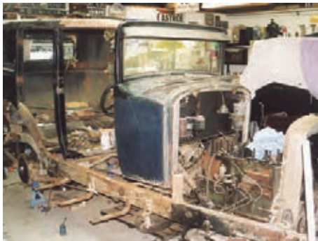
Body is lifted to enable floor repairs.
