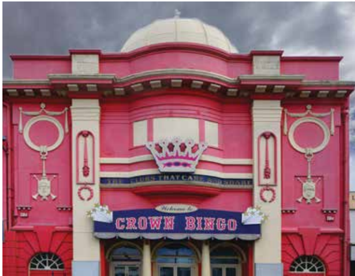
(top) Former Gaumont cinema, Fratton. Opened in 1928 and originally called the Plaza, it was the first cinema outside London to show a talking picture. It closed in 1965 and operated as a bingo hall until 1997, when it was converted into a mosque.
