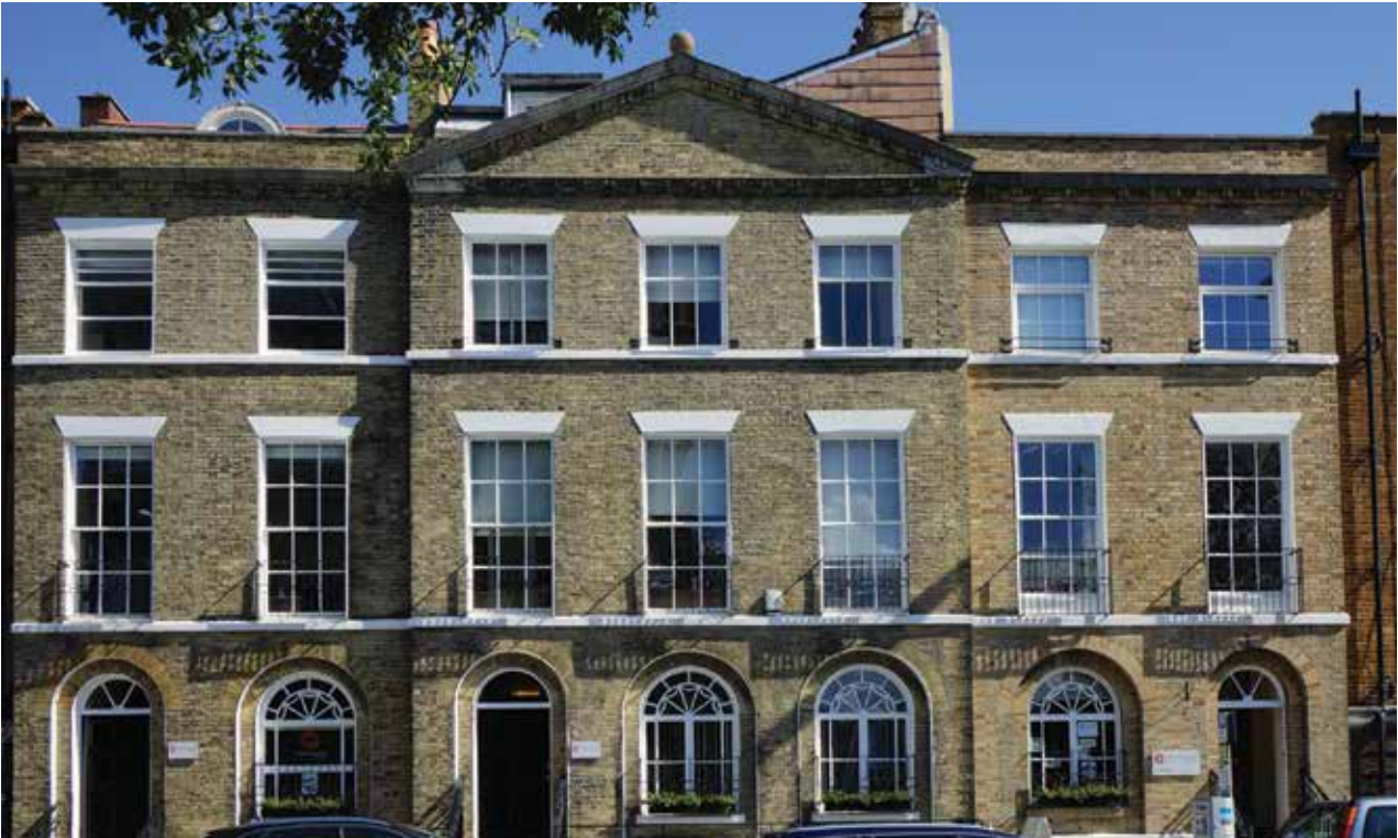
Kings Terrace. Built around 1810 to face newly-open ground created by the removal of the ravelins and walls of the old town defences.
