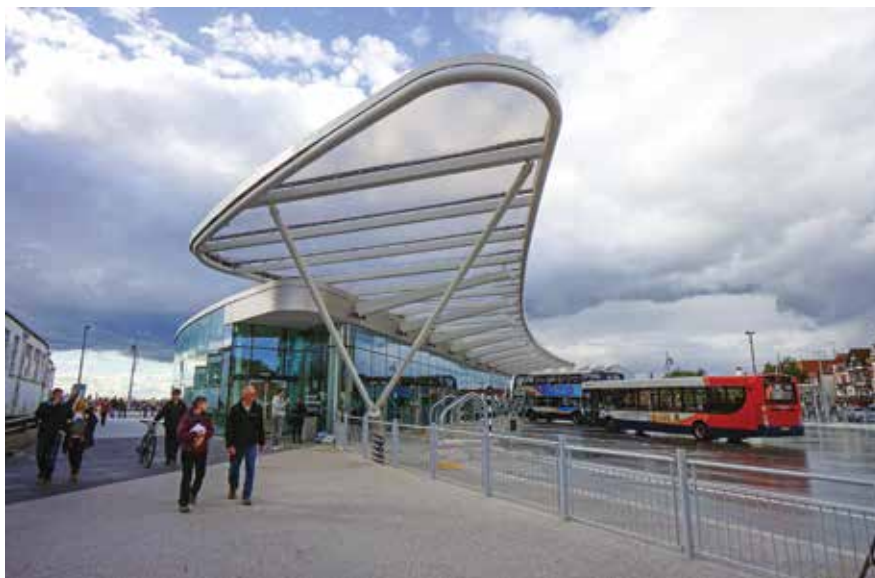
Transport Interchange, The Hard. The key element in the Council's plan for the regeneration of The Hard links bus and coach services with the Gosport ferry and Portsmouth Harbour train station.
