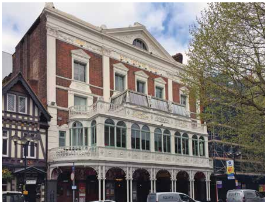
Theatre Royal, Guildhall Walk. Built as Landport Hall music hall in 1854, converted to a theatre in 1856, substantially rebuilt in 1884 and reconstructed by Frank Matcham in 1900.
