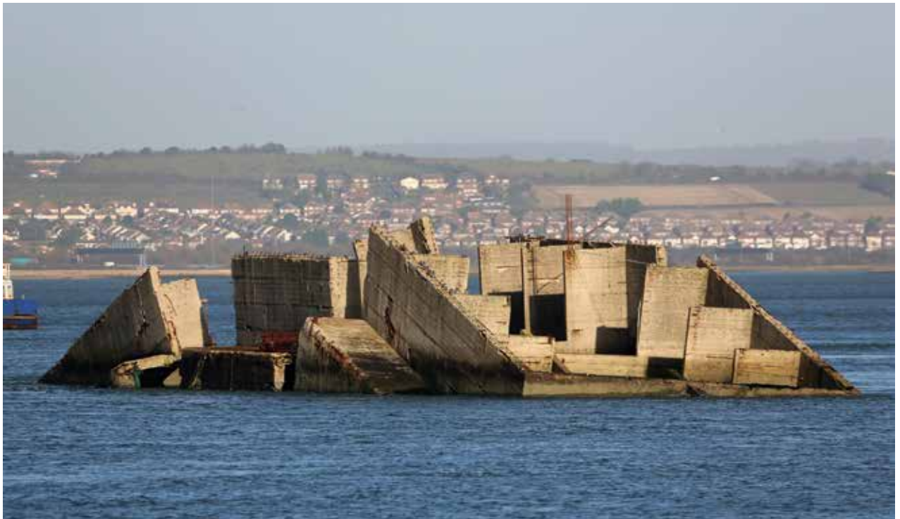
Mulberry Harbour wreck. The remains of a faulty Type C Phoenix Breakwater module, built on Hayling Island and designed to be part of the Mulberry Harbour infrastructure that was key to the D-Day landings in Normandy in 1944.
