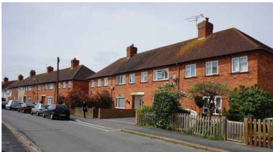
Hilsea Crescent, Hilsea. Council housing built in the late 1920s.
