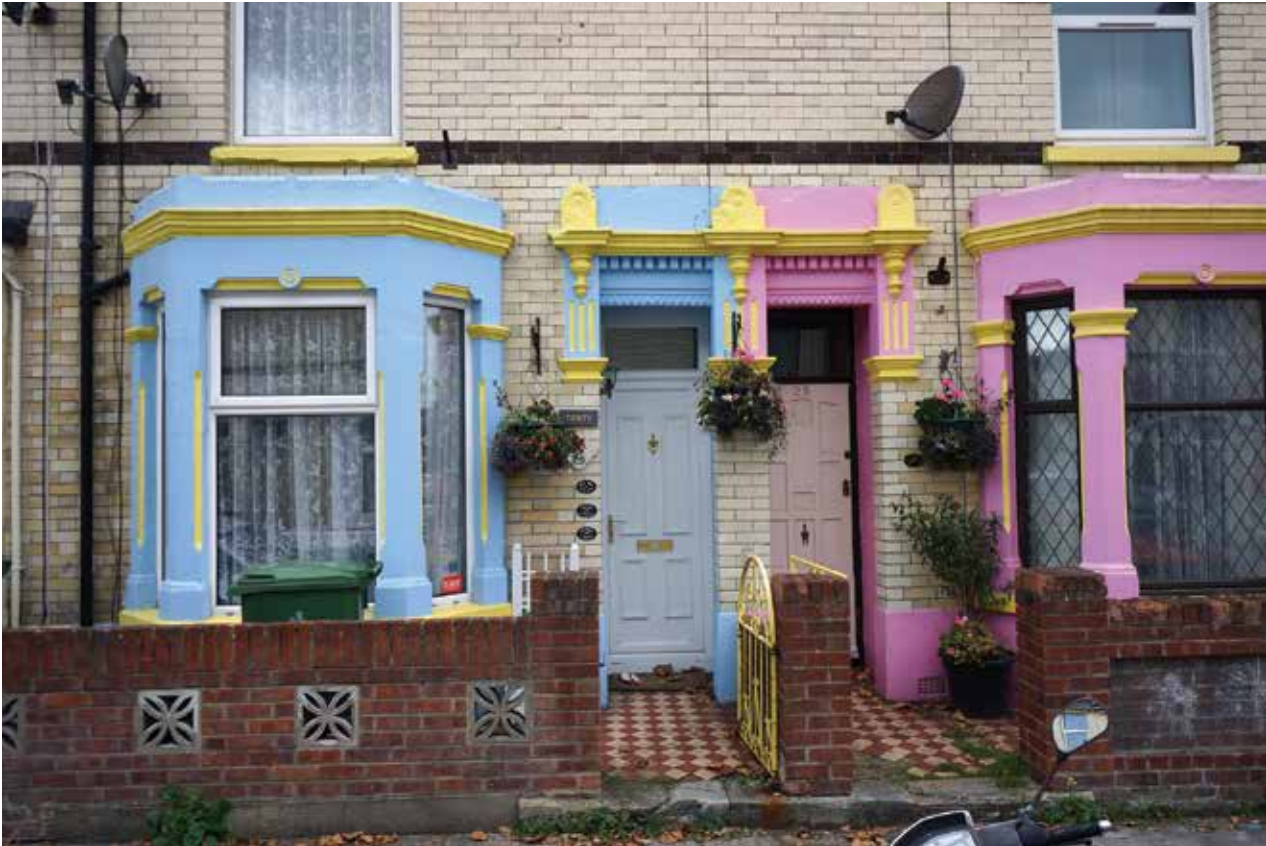
Burleigh Road, Fratton. Part of a Late Victorian terrace (1897) featuring the white tiled bricks deployed by speculative developers to lend a certain distinction to their product; the colours came later.
