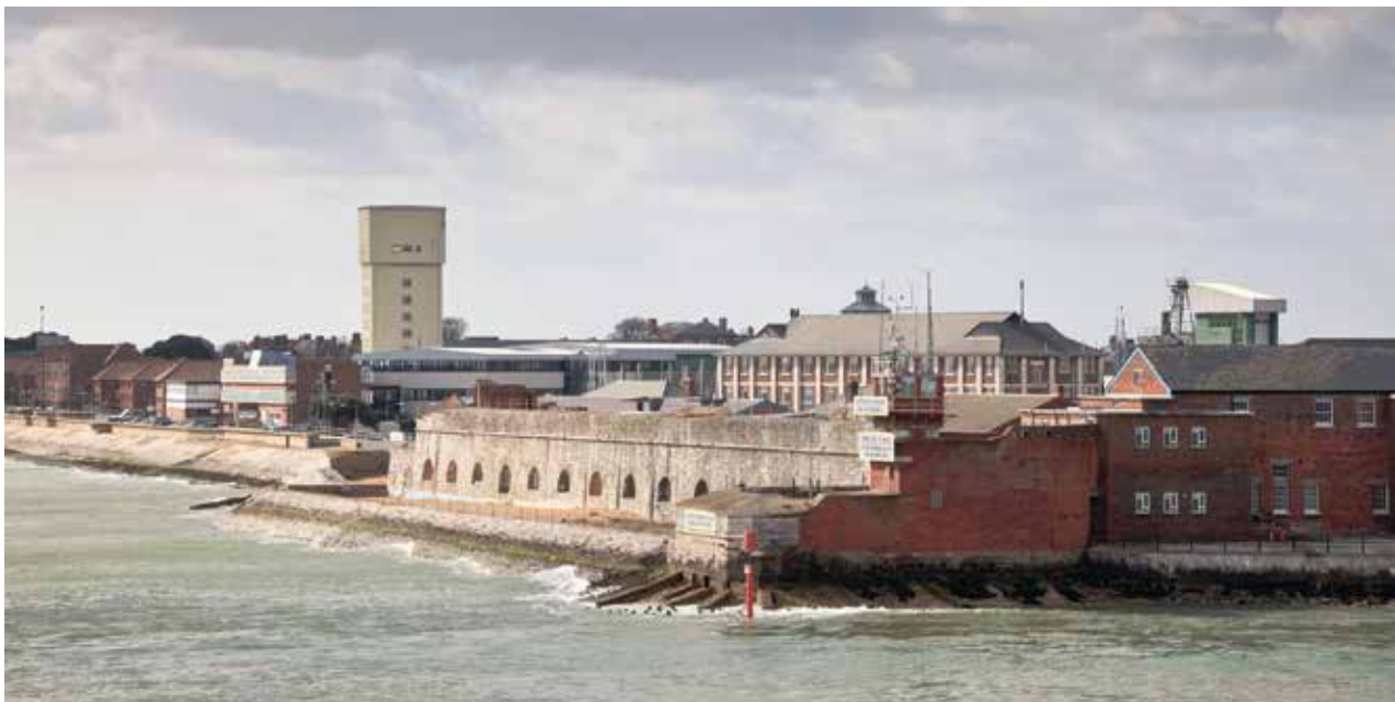
Blockhouse Point. Originally fortified in the fifteenth century, the stone battery dates from the 1660s and was subsequently incorporated into Fort Blockhouse.
