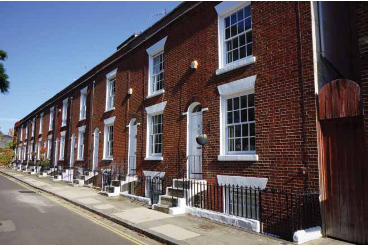
Gloucester View. This terrace of eleven small brick Georgian-style houses dates from the 1840s.
