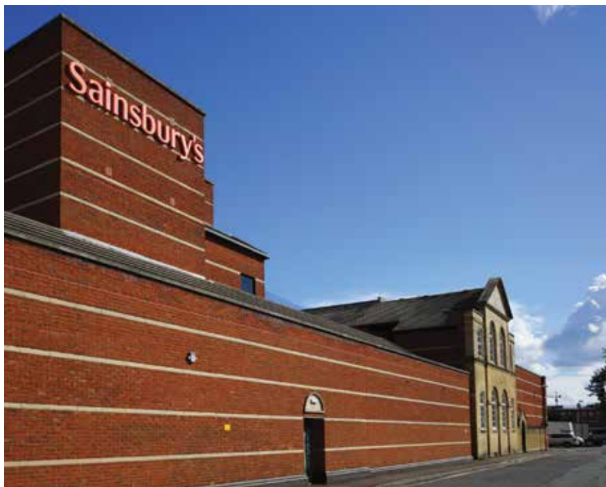
Sainsbury's supermarket, Clarence Street. The new building incorporates the facade of the Portsea Institution, formerly the Bell School (see page 51).
