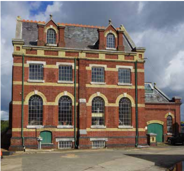
The Pumphouse, Eastney. Built in 1887 to house two compound beam engines by James Watt, the pumphouse was part of a state-of-the-art complex that included a boiler house and gas engine house.
