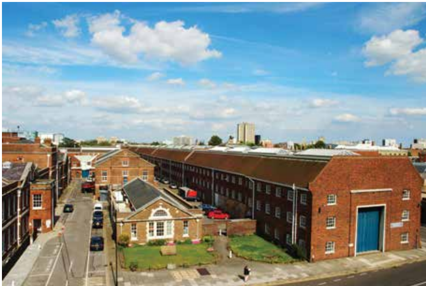
Ropehouse and Hatchelling House. In this long (1,095 feet) 3-storey structure, built in 1771, hemp was straightened out, or hatchelled, before being made into hemp strings, which were then spun into rope. To the left of the Ropehouse in the photo is the Tarring House (1747).
