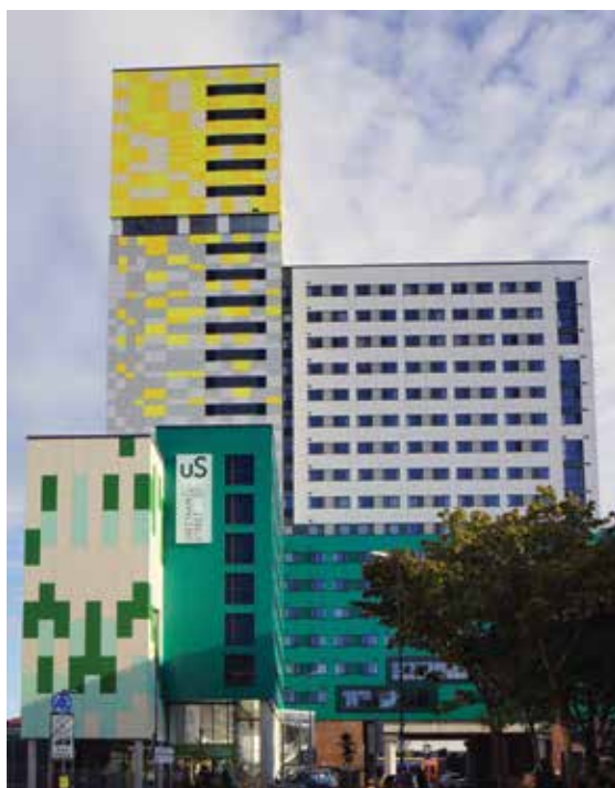
Unite Students Building, Greetham Street. Designed by Cooley Architects for Unite, the biggest student housing provider in the country. Completed in 2016, just in time to make the shortlist for the 2017 Carbuncle Cup, awarded by Building Design magazine for Britain's ugliest new building.
