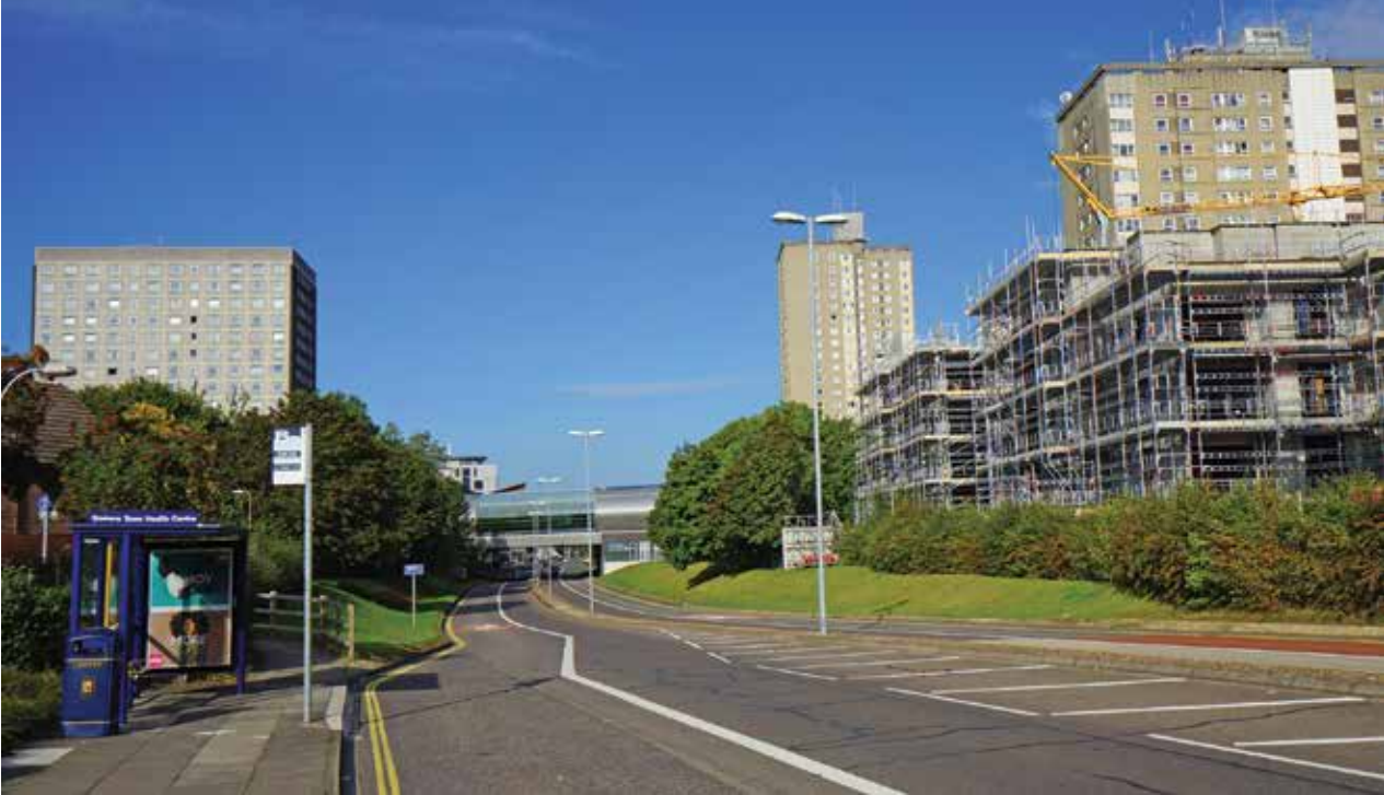
Winston Churchill Avenue, Somerstown. Created in the early 1970s as a key east-west route across the city, it cut Somerstown in two, with few safe crossing points.
