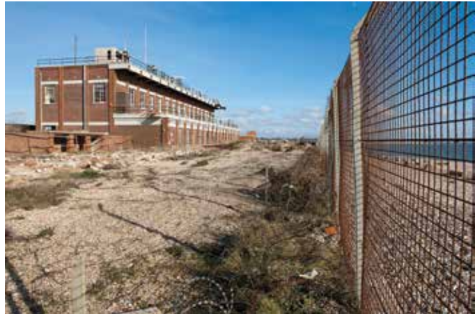
Fraser Range, Eastney. One of the few remaining sites available for development on Portsea Island, the former Royal Navy gunnery school has been sold for residential development.
