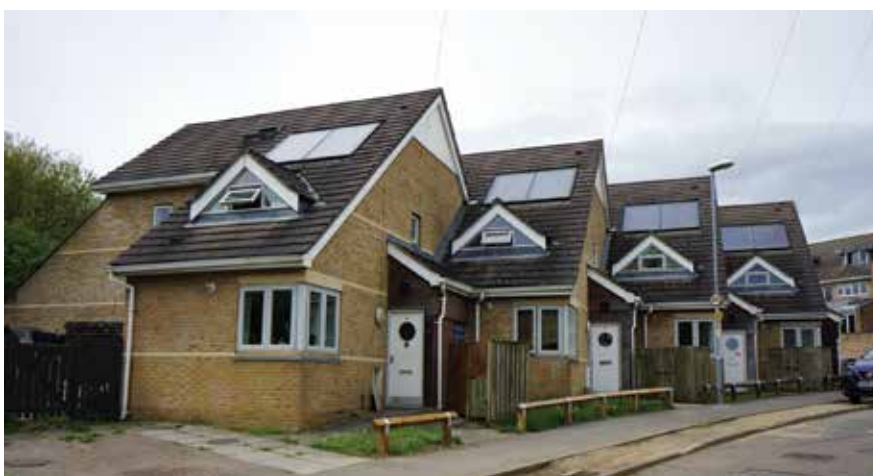
Jamieson Terrace, Paulsgrove. Eco-friendly, energy efficient social housing built in 2004.
