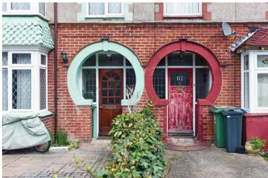
Chatsworth Avenue, Highbury. Built between 1934 and 1936, the estate consists of repeated terraces of six, 2-storey, dwellings with large distinctive arches above their front doors, tile-hung bay windows, and decorative boundary walls.
