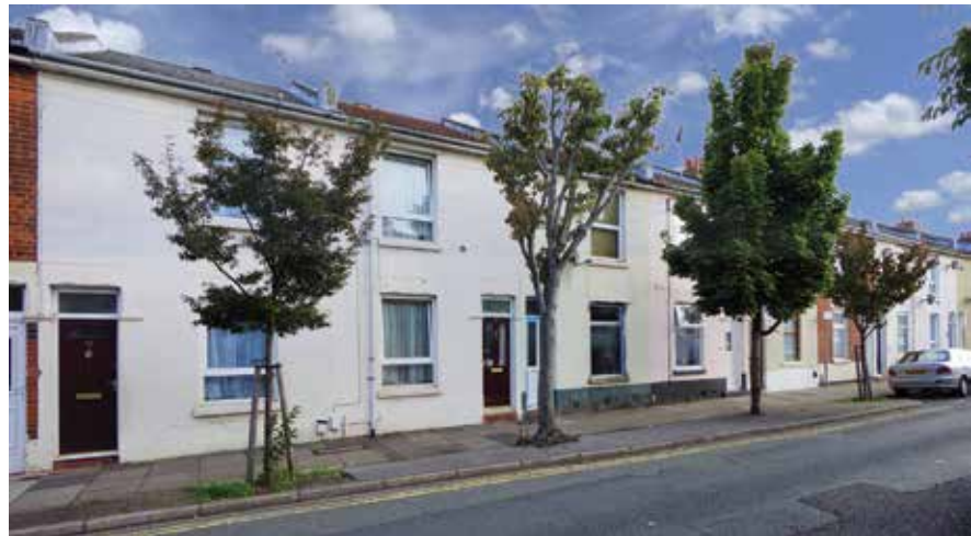
Lower Derby Road, Stubbington. One of Portsmouth's oldest surviving terraced streets, dating from the 1860s.
