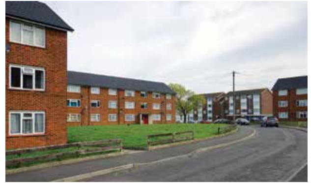
Naval housing, Eastney. Married quarters for naval ratings, built in the mid-1960s on the landfill of the Glory Hole.
