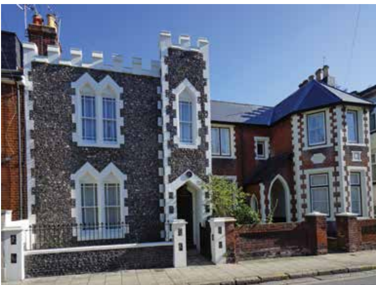
Stanley Street, Southsea. A pair of flamboyant houses built 1840-50, infilling the southern extension of T.E. Owen's Southsea developments.
