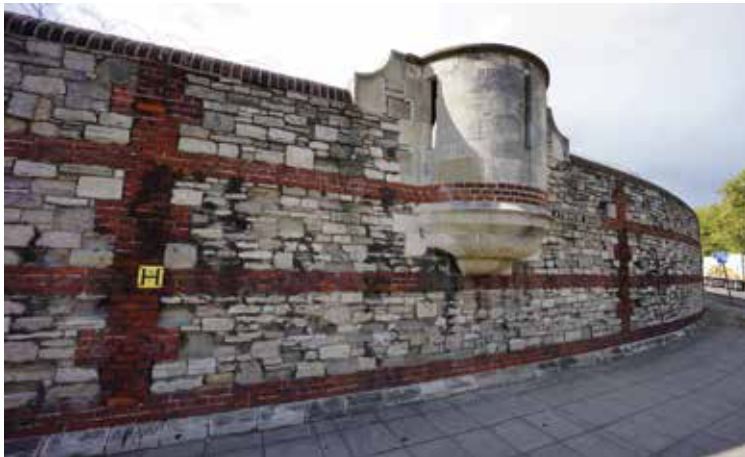
Dockyard Extension Wall. The 180-acre Great Extension programme that began in 1864 was enclosed with a new wall with oriel gun bastions, each with three gun slits.
