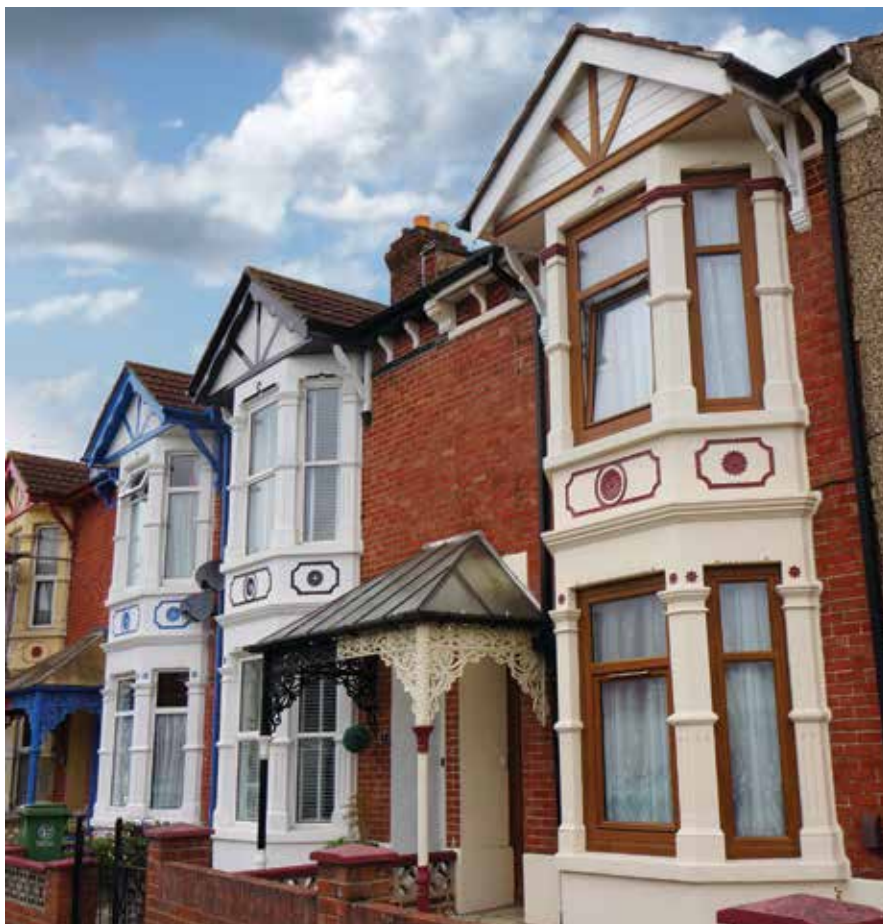
Tangier Road, Copnor. An Edwardian terrace featuring the wrought-iron porches that had proved popular in Victorian Southsea.
