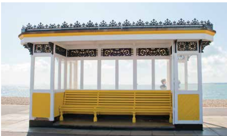
Seafront shelter. One of several surviving shelters erected along the seafront by the Council in 1903.
