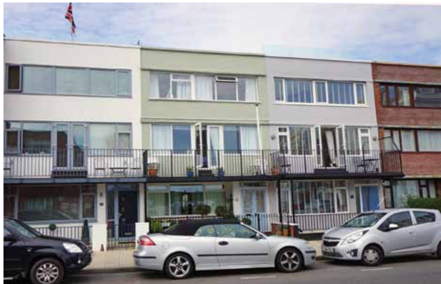
Maisonettes, Old Portsmouth. Replacements for bombed-out housing on High Street, they were a harbinger of the gentrification of Old Portsmouth.
