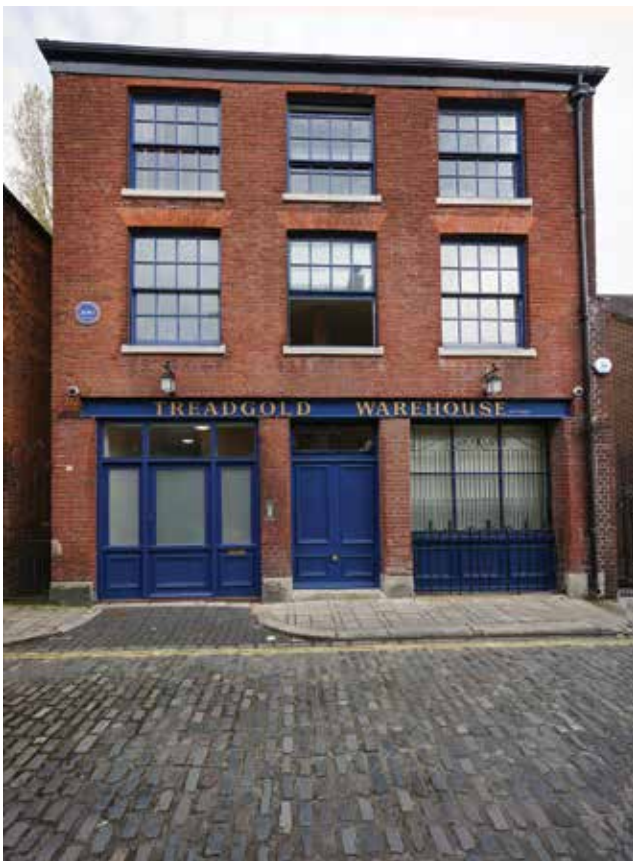
Treadgold's warehouse, Bishop Street.
