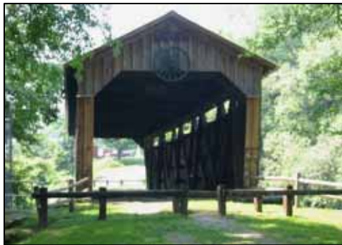
Kidd's Mills Covered Bridge
