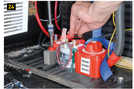
23) A weatherproof 50-amp breaker is used between the solar-panel connector box and the charge controller. 24) A master cutoff switch is used between the battery bank and the inverter and charge controller. Next to the switch is a solenoid that is triggered by the master BMS control. If any one cell falls below or exceeds the voltage threshold, it cuts off power from the battery bank.
