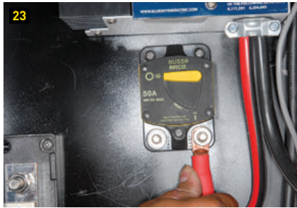
23) A weatherproof 50-amp breaker is used between the solar-panel connector box and the charge controller. 24) A master cutoff switch is used between the battery bank and the inverter and charge controller. Next to the switch is a solenoid that is triggered by the master BMS control. If any one cell falls below or exceeds the voltage threshold, it cuts off power from the battery bank.
