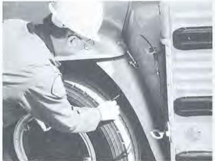
Inspecting school bus steering and tire tread depth.
