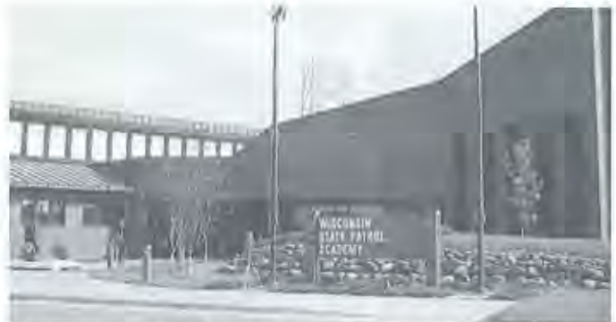
The new State Patrol Academy provides training to law enforcement officers from state, county and municipal agencies.
