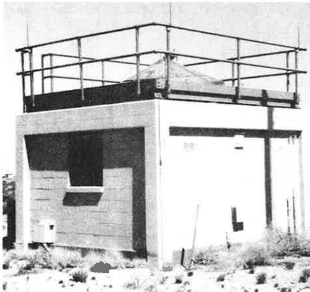
The Mitchell camera building at C Station, facing northeast.
