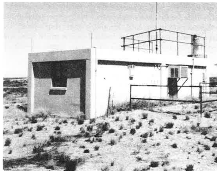
The double Askania cinetheodolite building at C Station, facing northeast.
