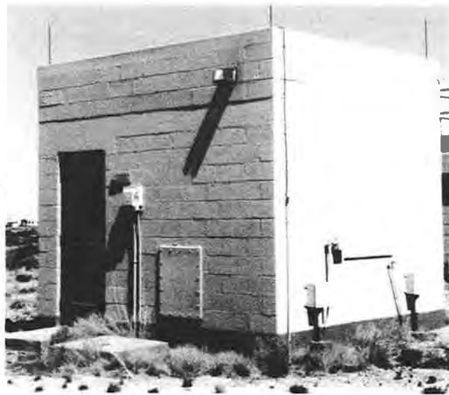
The impact predictor building at C station.
