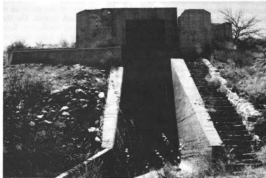
The 100-K static test stand, capable of testing up to 100,000 pounds of thrust.
