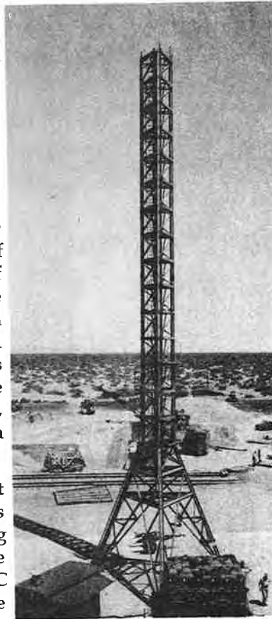
WAC Corporal launcher at LC-33, no date. Gantry crane track installation in background (Sauber photo from private collection).
