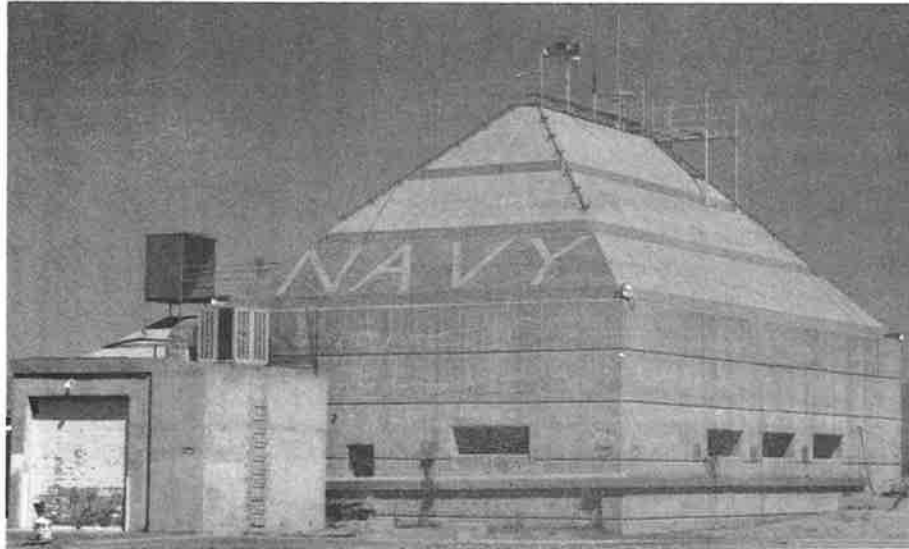
The Navy blockhouse at LC-35 (Army Launch Area 2), 1995.
