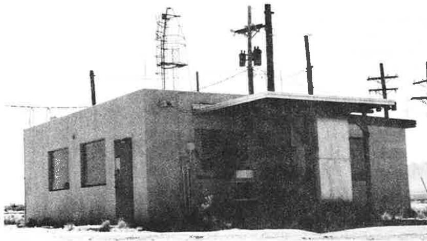
The telemetry building at C Station.
