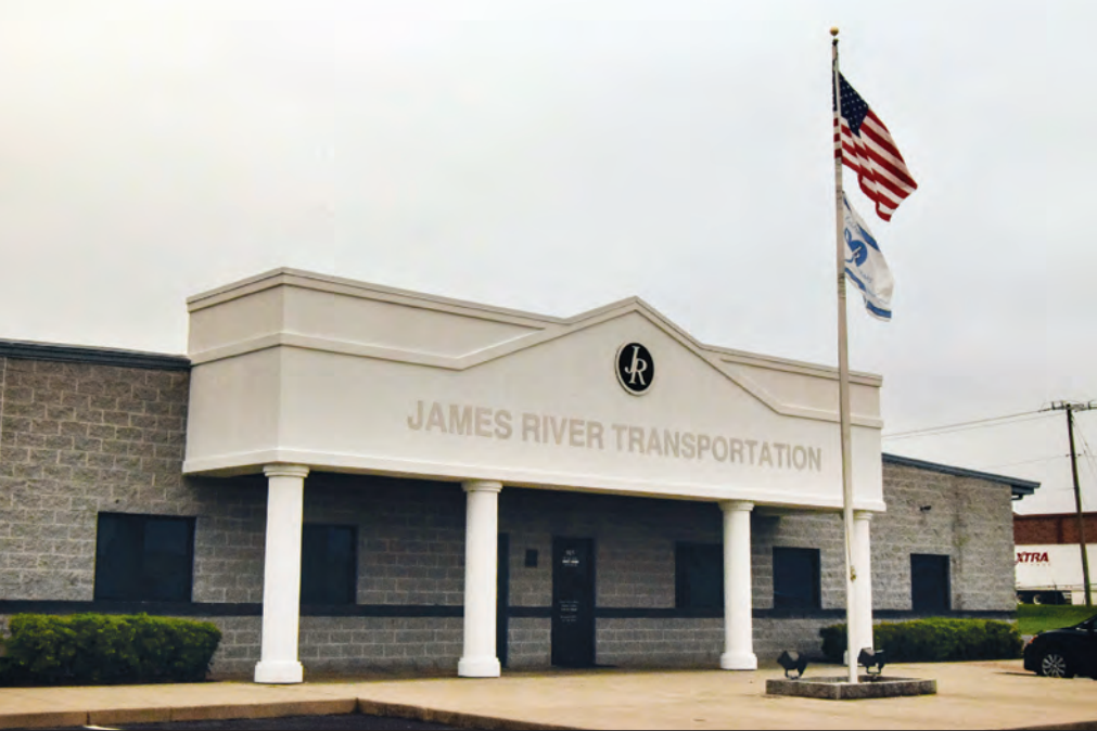
The main facility of James River Transportation, located in Richmond, VA, was built in 1998.
