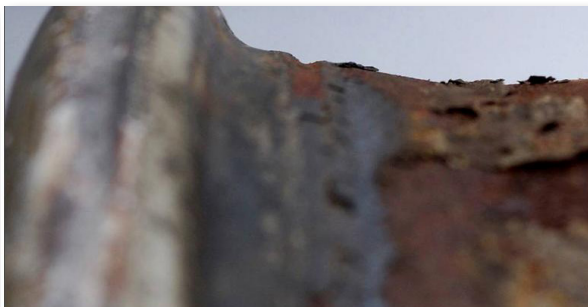
Wear on the seat due to corrosion and overloading
