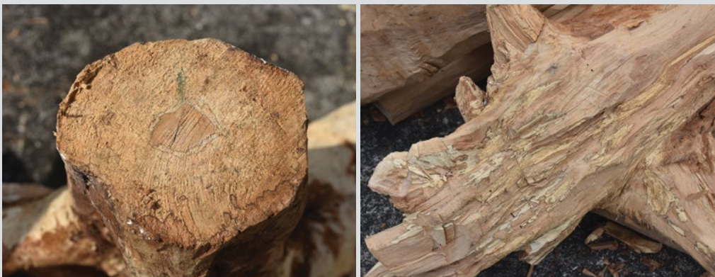
Figure 10.11 Rotten wood – heartwood with significant areas of degradation associated with water or disease entry into the wood
