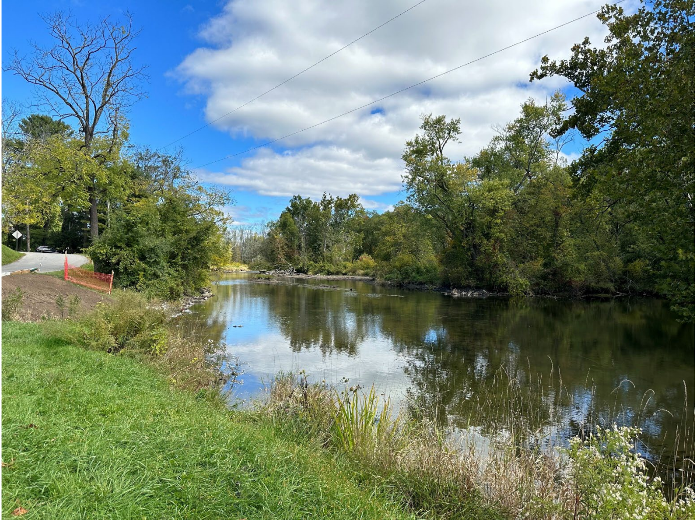
County Line Dam Removal Site (After), Paulins Kill, NJ; Photo Credit: The Nature Conservancy
