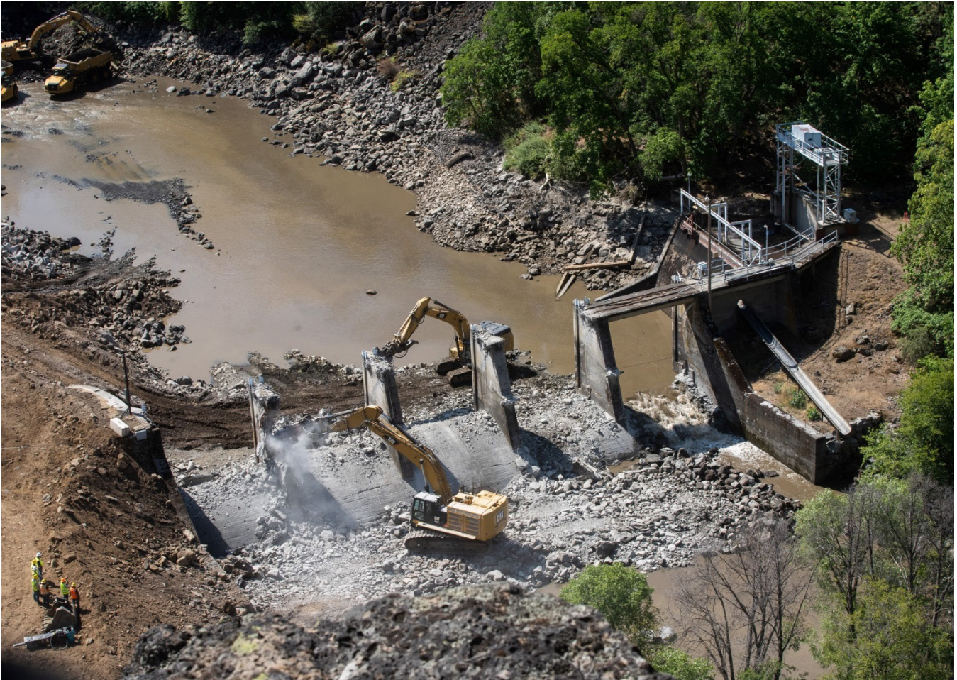
Copco 2 Dam, Klamath River, California Credit: Swiftwater Films
