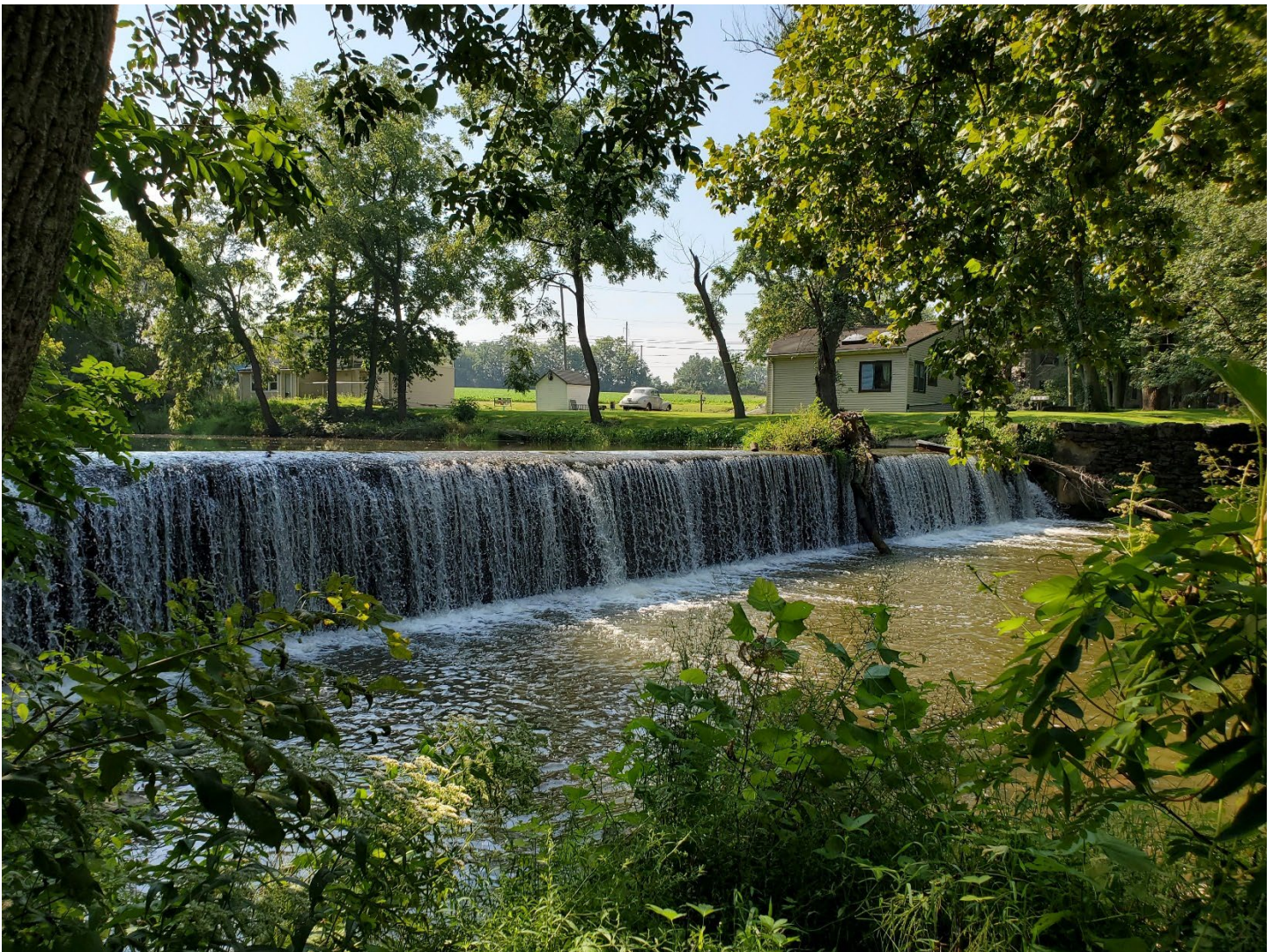
Chiques Roller Mill Dam, Chiques Creek, PA; Photo Credit: Jessie Thomas-Blate
