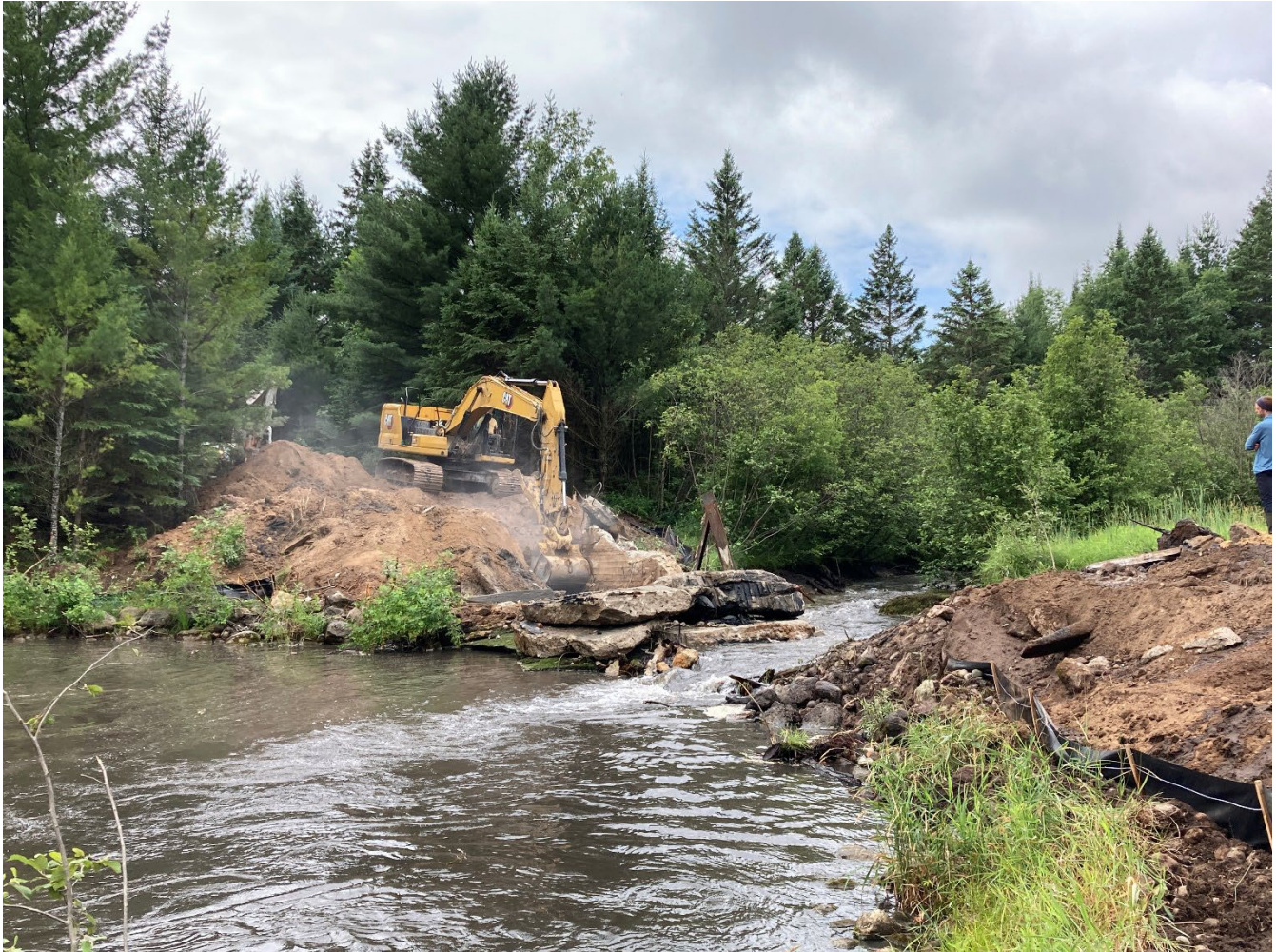
Timberland Dam, West Branch Tittabawassee River, Michigan Credit: Huron Pines
