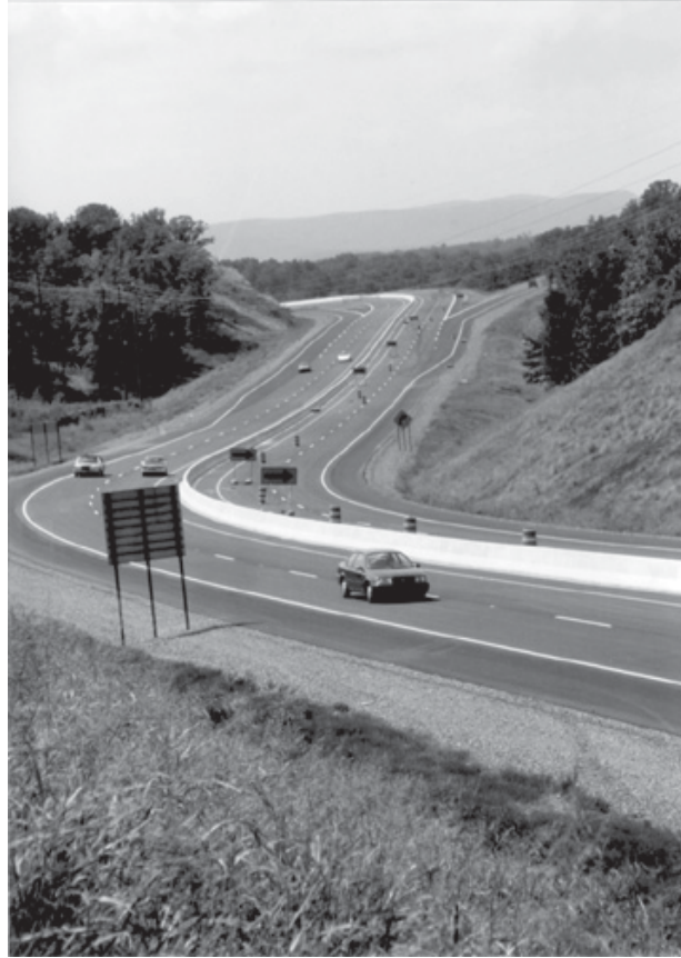
The first leg of the East-West Arterial linking Highway 270 West and Highway 70 West in Hot Springs.
