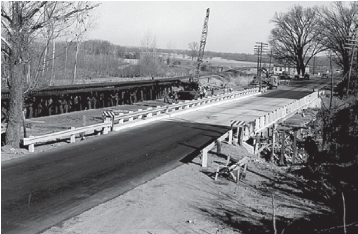
The widening of Palarm Creek Bridge on Highway 365 in 1956.
