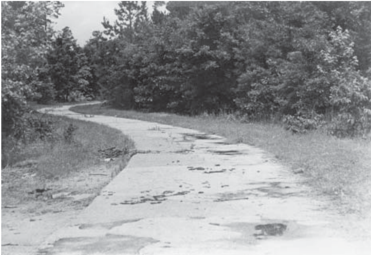
Dedicated in 1914, the Dollar Way Road, extending northwest from Pine Bluff to the Pulaski County line, was the longest continuous stretch of concrete pavement in the nation. Total cost was $158,000 for the 23.6 miles of pavement, or approximately $1 per lineal foot; thus the name "The Dollar Way."
