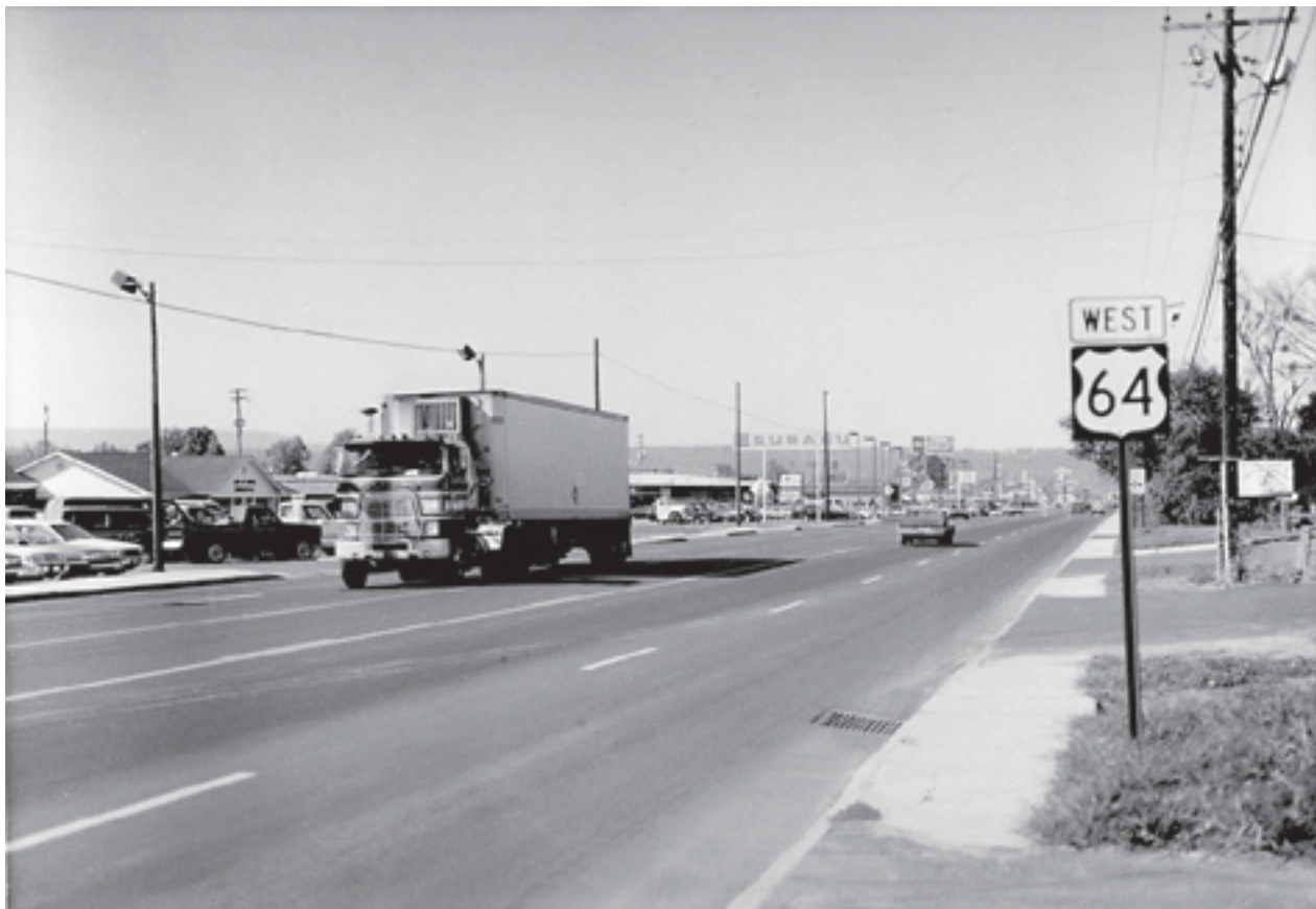
A five-lane Highway 64 at Russellville.
