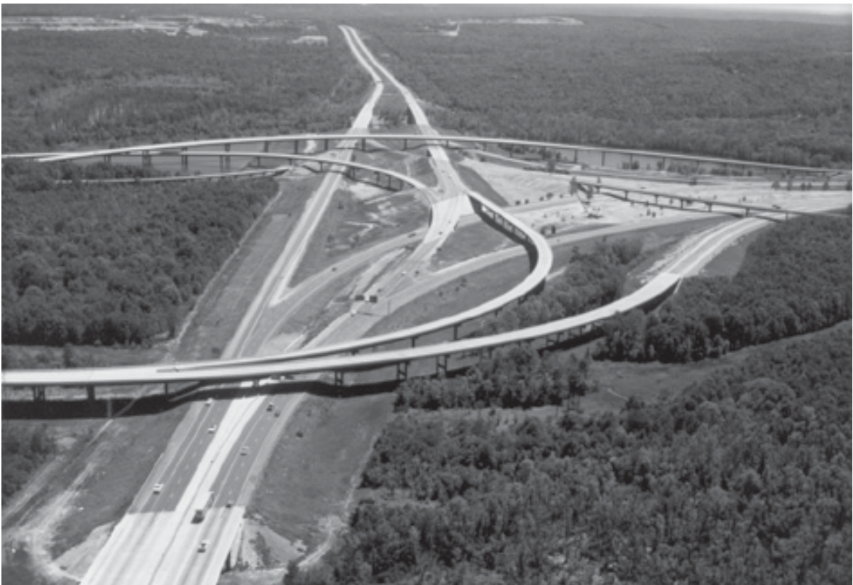
The South Terminal Interchange of I-30, Highway 65 and I-440 in Little Rock.
