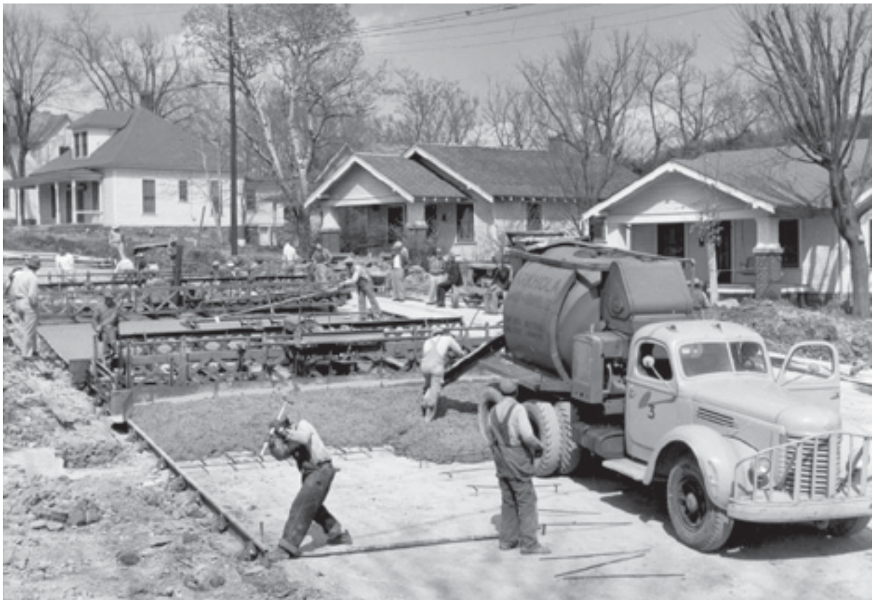
Construction on Highway 71 at Fayetteville in 1952.
