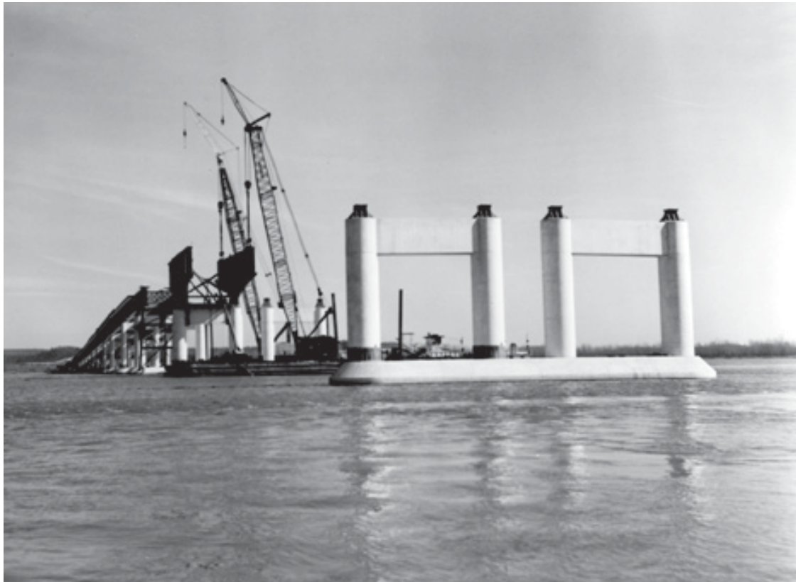
The Interstate 430 Arkansas River Bridge under construction in 1973.
