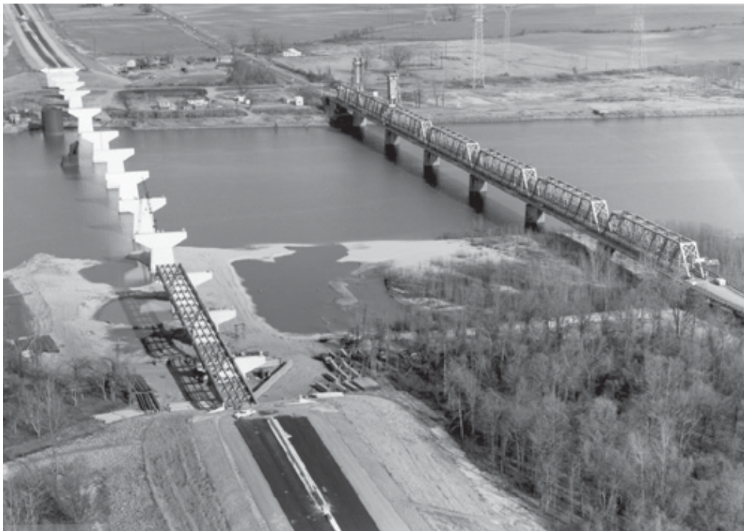
The Highway 79 Arkansas River Bridge under construction at Pine Bluff in 1970.
