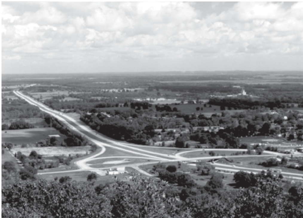
Interstate 40 and Highway 105 Interchange at Atkins in Pope County.
