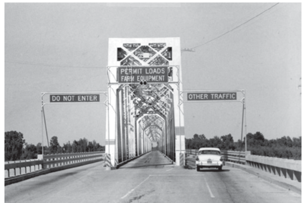
Arkansas River Bridge on Highway 79 at Pine Bluff in 1956.
