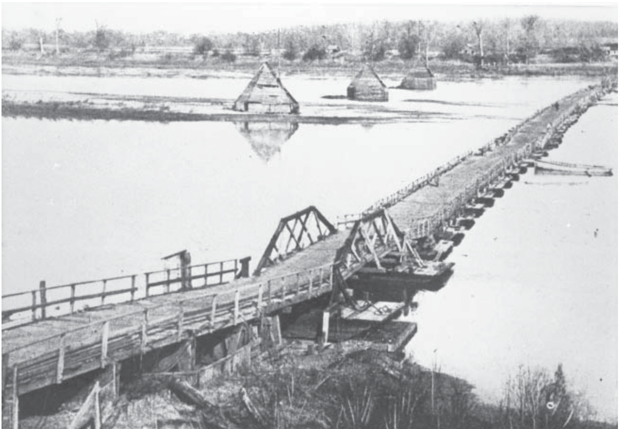
The 2,208-foot pontoon bridge over the Arkansas River at Dardanelle, said to be the longest bridge of its kind in the world at that time, was constructed in 1890 as a toll facility. The pontoon bridge was replaced in 1929 by a steel structure, passable at no charge.
