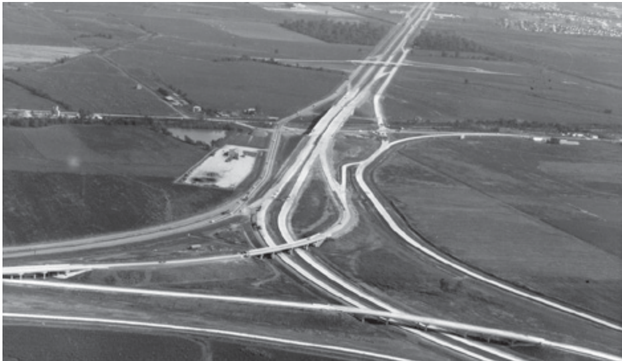
Construction on the Interstate 55/Interstate 40 Interchange at West Memphis in 1960.
