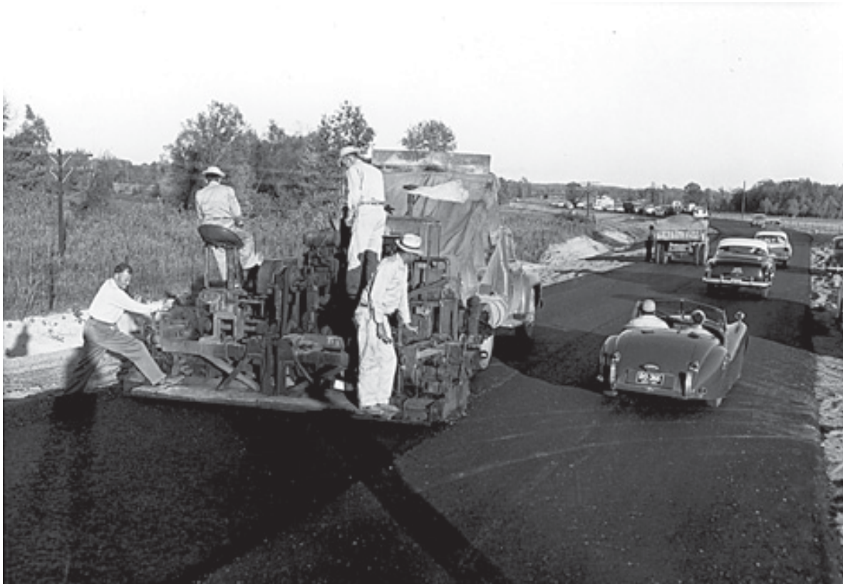
The widening of Highway 67 south of Malvern in 1956.
