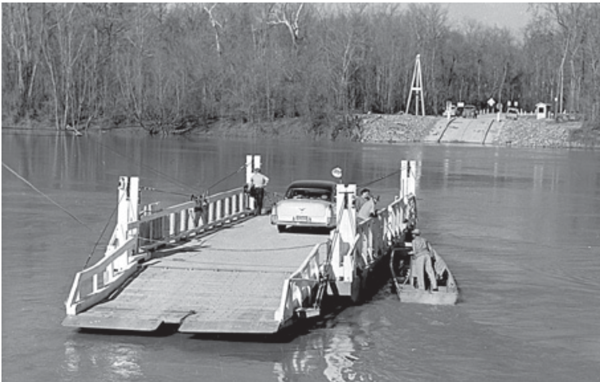
The cable-operated St. Charles Ferry crossed the White River at Highway 1 for 27 years before it was taken out of operation in December 1981.
