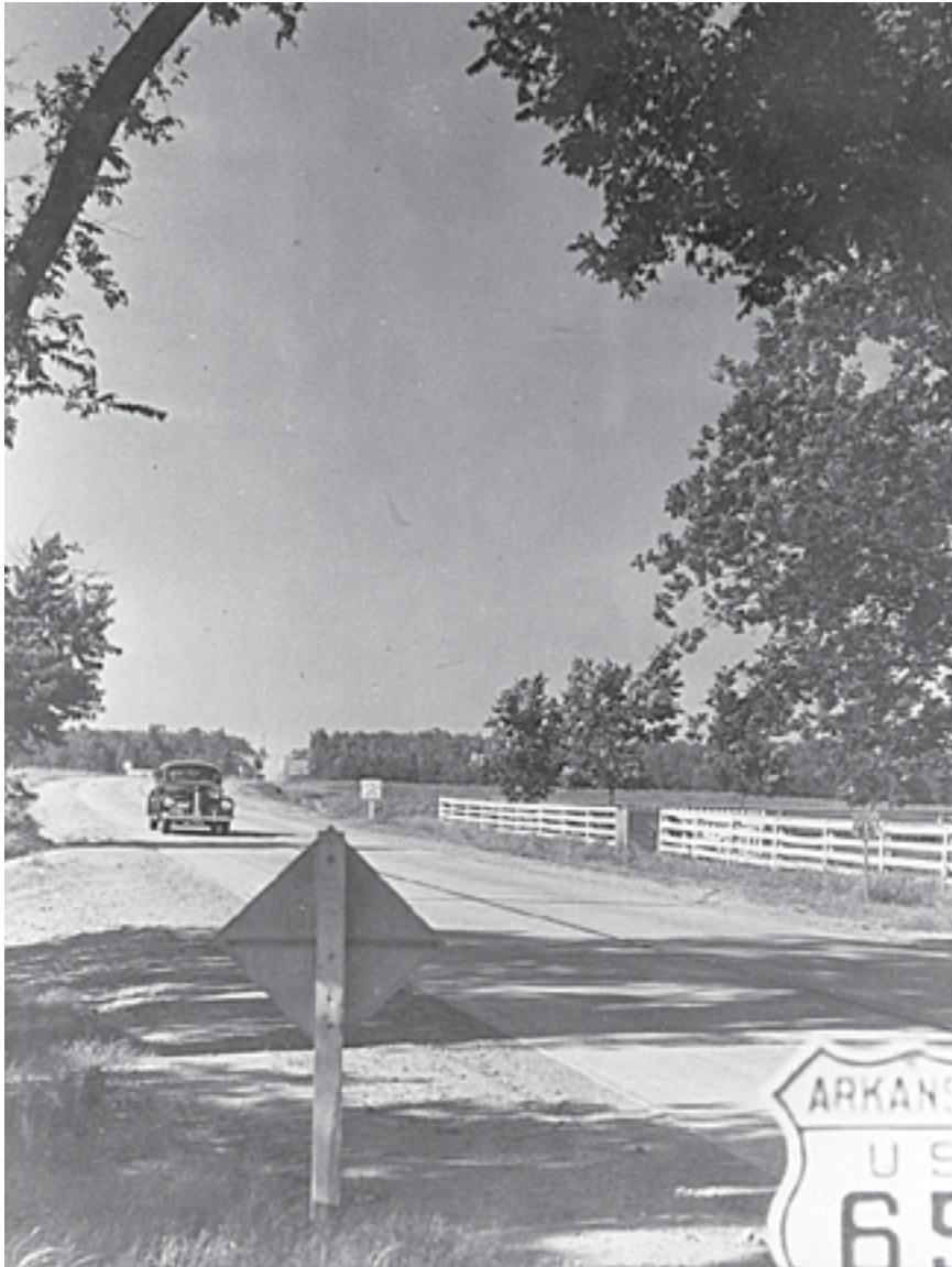
Highway 65 at Palarm Creek at the Faulkner-Pulaski county line.
