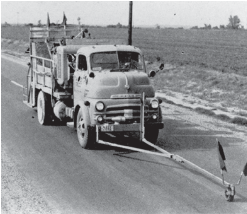
Centerline striping on Highway 11 near Stuttgart.
