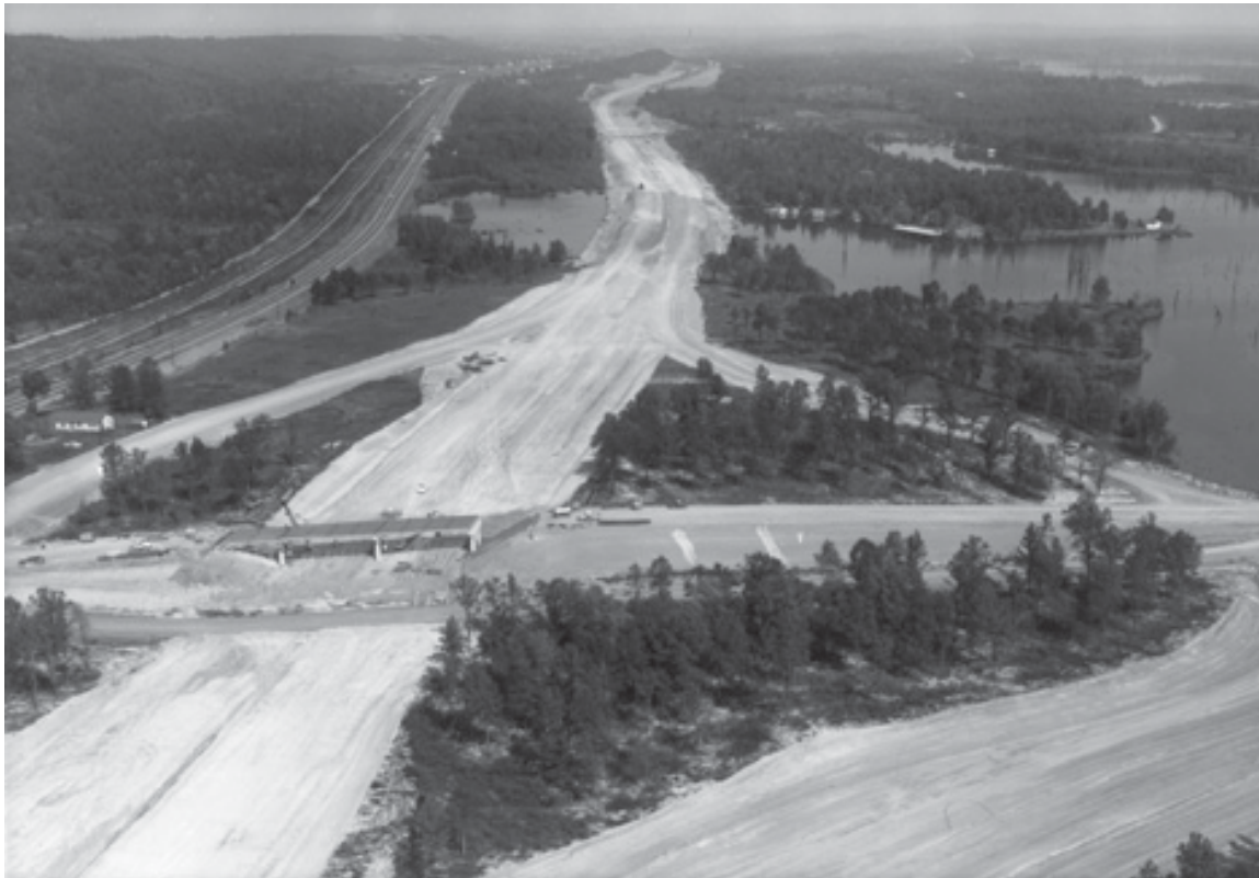
Construction of Interstate 40 at the Highway 89 (Mayflower) Overpass in 1965.
