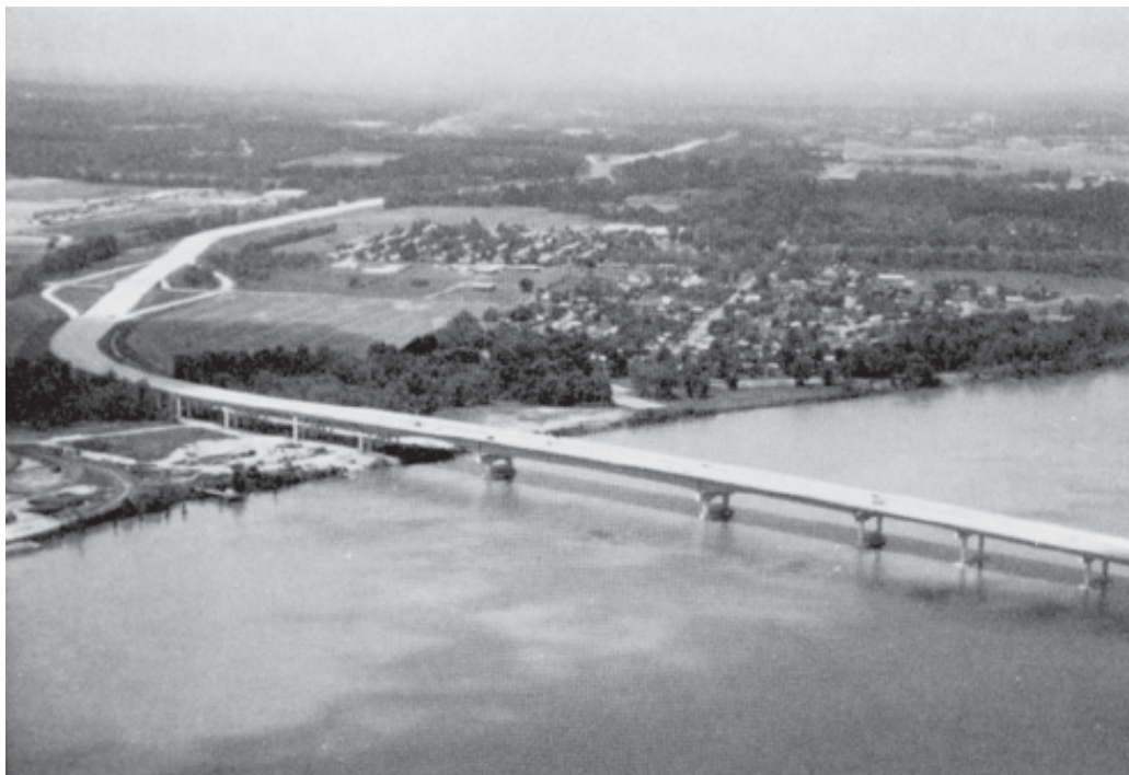
The Interstate 440 Bridge across the Arkansas River at Little Rock.
