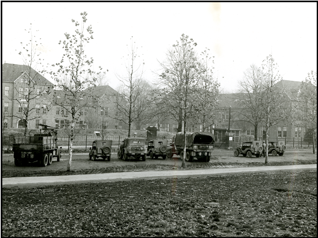
Figure 5.4. Combined Ninth Army and XXIX TAC Headquarters, Maastricht, Netherlands.
