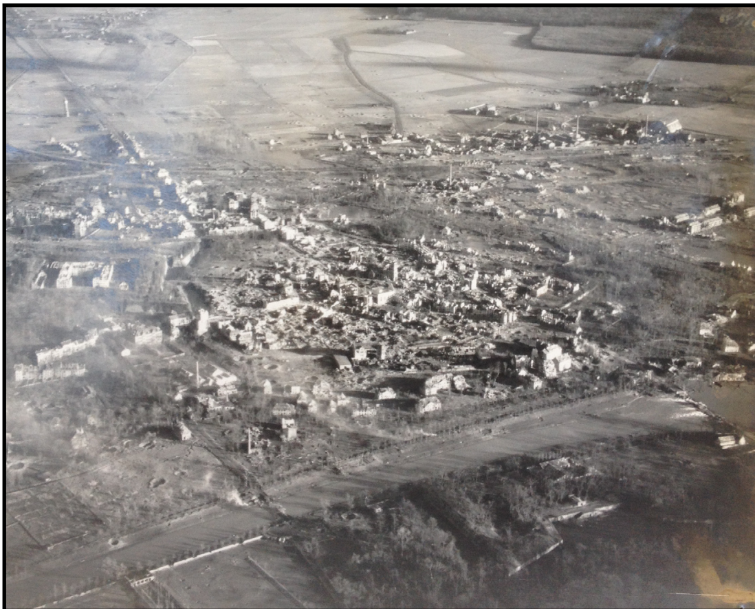
Figure 5.3. Bomb Damage in Julich during Operation Queen.
