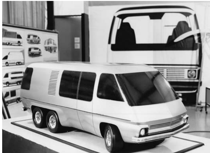
During the GMC Motorhome design phase, clay models were created to test different ideas, among them the 1/8-scale model above, shown with a full-size tape drawing and various sketches in the background. These led to the production of a full-size clay model, known as RV-26 (pictured top and bottom); note the wraparound taillights and rear window styling of this model.
