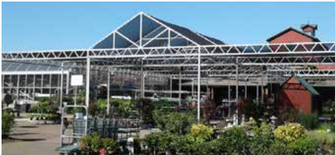
Peaked Roof W-Truss
