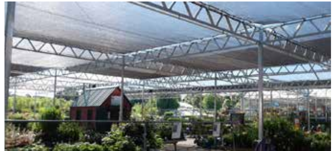
Standard Roof W-Truss
