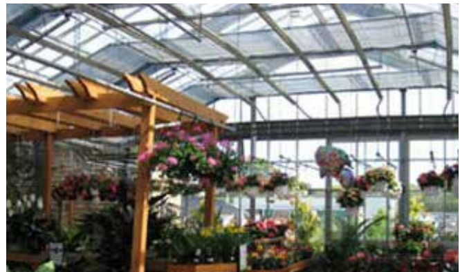
Dual curtain system (shade and blackout).
