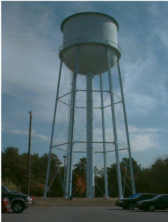
World War II water tower
