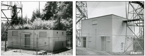
Figure 5. Type 1600 Chehalis Microwave Radio Station Building, 1950 (left, NARA:ChehalisMWNARABox17-008).Two-story Early Modern Type 1602 Building at Squak Mountain Microwave Radio Station, 1951, (right, NARA:Squak2NARAbox27of52-014).
