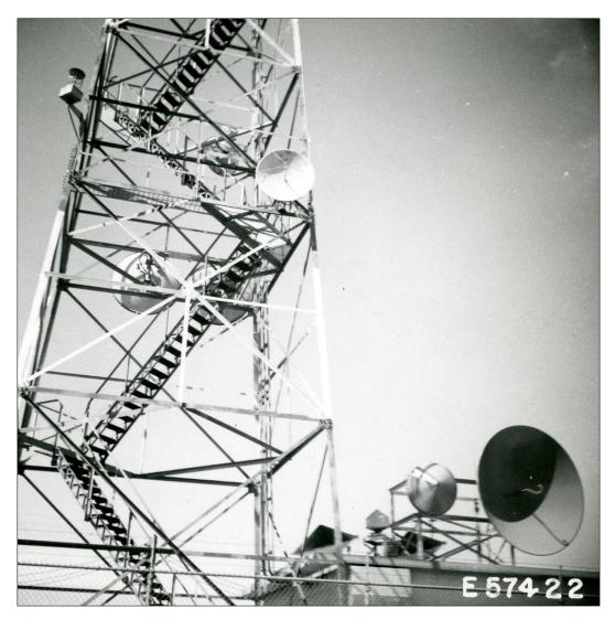
Figure 13. Four-leg Steel Lattice Tower with Internal Staircase at Beverly Microwave Radio Station, nd. (NARA:BeverlyMWNARAbox10-013).
