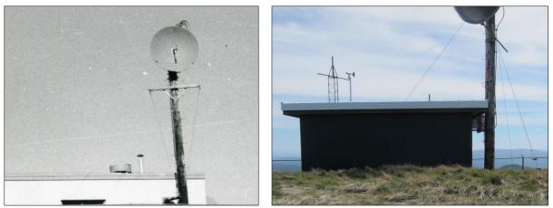
Figure 15. Wood monopole tower at Mary's Peak Microwave Radio Station in 1960 (left, NARA: MarysPeakNARAbox16of52-005, cropped) and 2019 (right).
