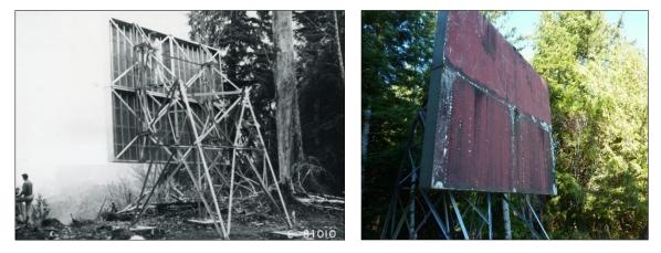
Figure 16. Driscoll Passive Repeater in 1967 (left, NARA: DriscollNARAbox26-005) and c. 2016 (right).
