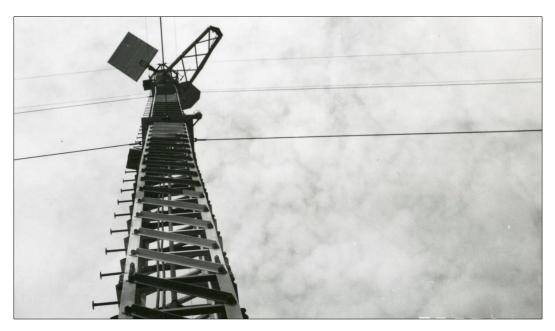
Figure 14. Four-leg steel Lattice Tower with Guyed Wires at Leneve Microwave Rado Station, 1961 (NARA:LeneveNARAbox15of52-003).
