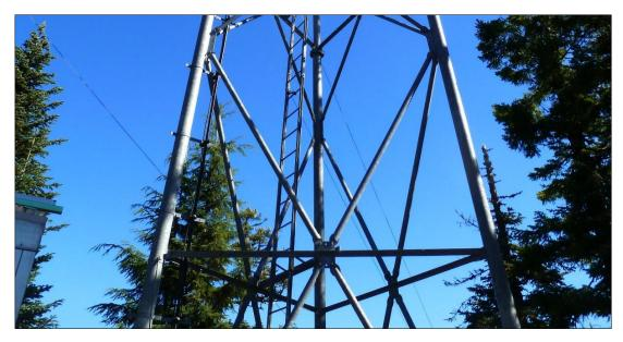
Figure 12. Three-leg Steel Lattice tower at Hall Ridge Microwave Radio Station.
