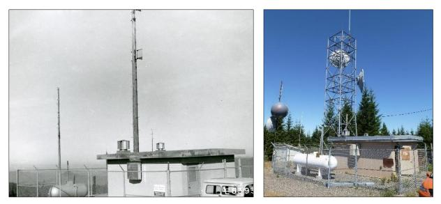
Figure 17. Kenyon Mountain Microwave Radio Station original monopole antenna tower circa 1960 (left, NARA:KenyonNARAbox14of52-002); replacement four-leg lattice steel antenna tower circa 2012 (right).
