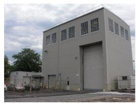
Figure 48. The Midway Untanking Tower with its original distinctive door retains overall integrity, while the new roll-up door diminishes the integrity of the Bell Untanking Tower.
