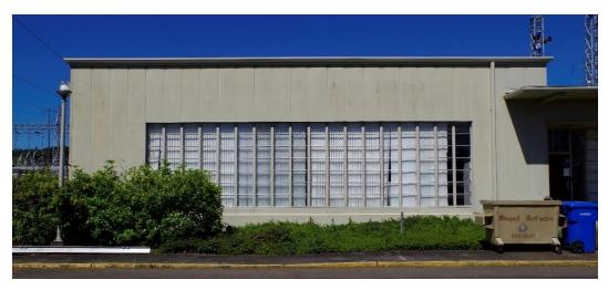
Figure 50. Alvey Control House with steel windows
