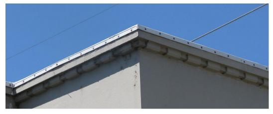
Figure 56. Midway Control House Dentils Detail
