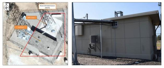
Figure 18. Penetration of the north wall of the Waterville Station Building to bond the ground bar to the outside grounding.
